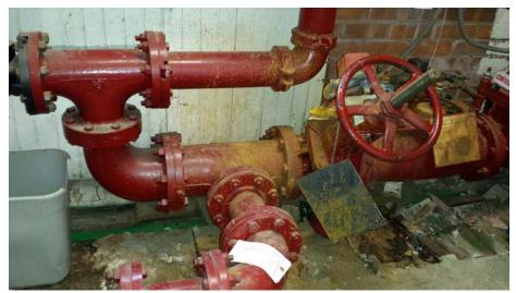
Recommendations: Verify history and source of the moisture and staining. Assure that all major test/drain piping is directed outside and drains adequately away from the building. Assure all minor/auxiliary drain piping that cannot drain by gravity to outside is directed to a viable drainage system.
