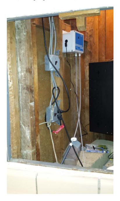
Toggling the switch on and off had no apparent effect on the fan's very low air flow, and the pump did not operate, presumably because pump start/shutoff is controlled through liquid level sensing.
