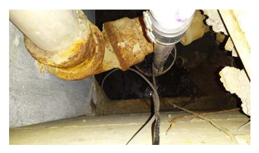
Pump discharge was piped into a storm main dropping to below grade in the same wall cavity.
