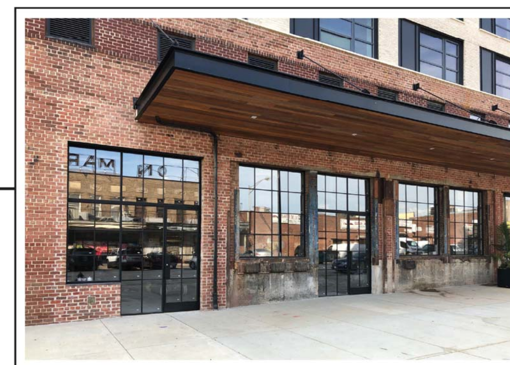
METAL CANOPY & STOREFRONT WINDOWS
