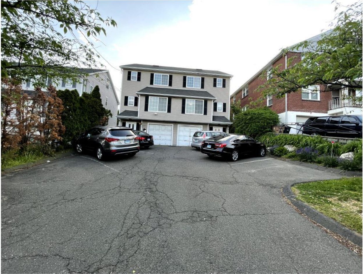
Front of property/off-street parking
