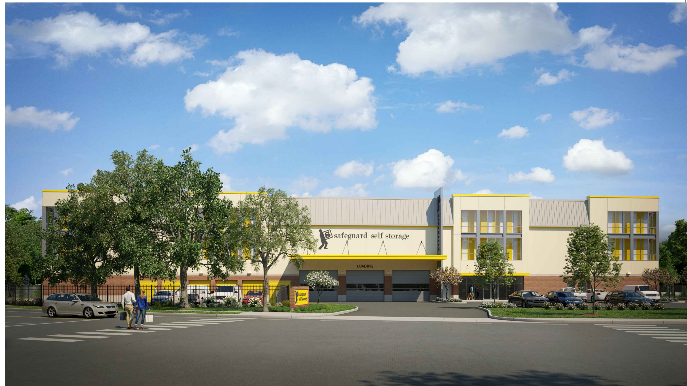
3 LOOKING EAST ON TOMS ROAD - NEW SCALE: N.T.S.
