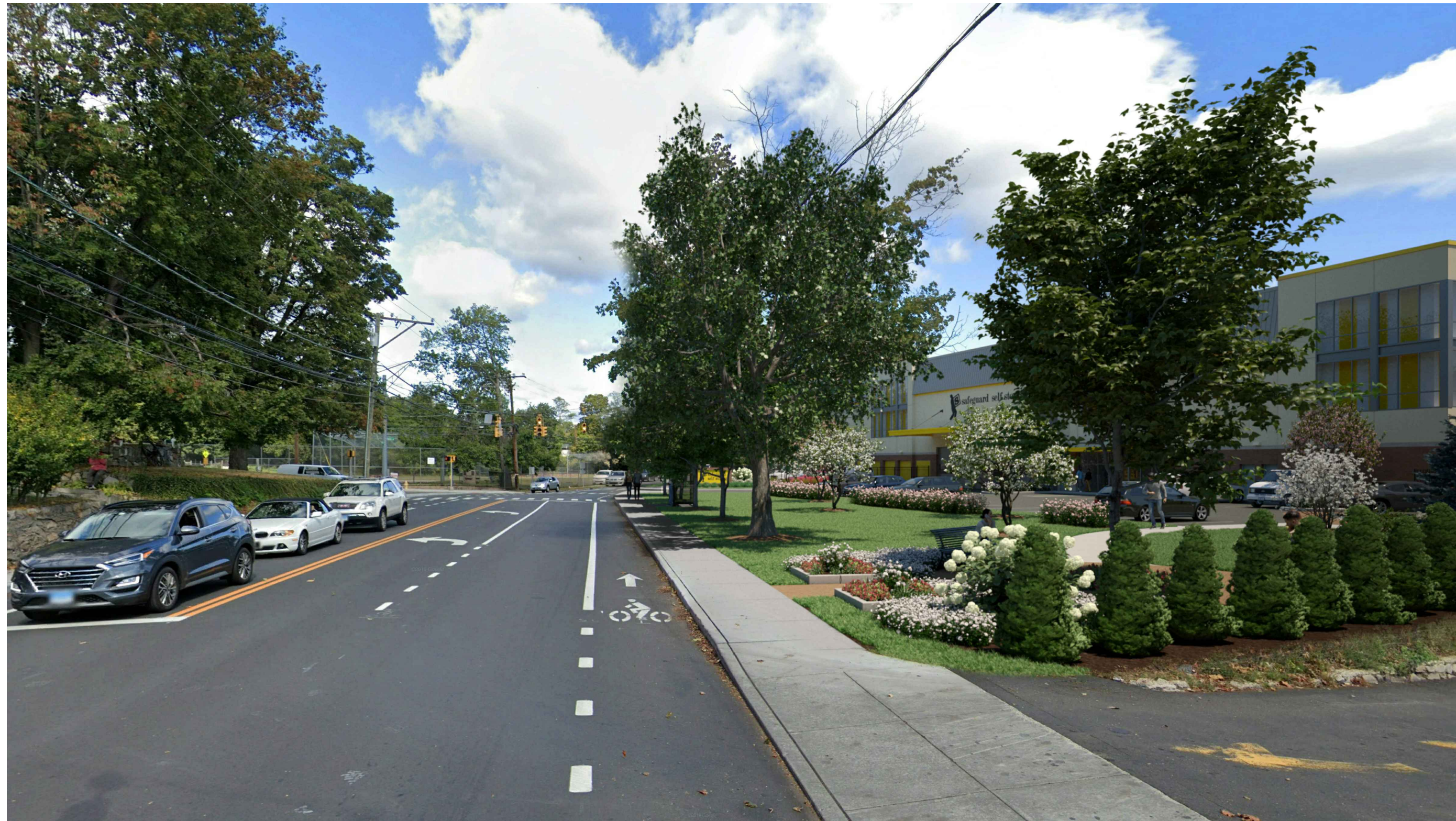
4 LOOKING NORTH ON HOPE STREET - MATURE SCALE: N.T.S.
