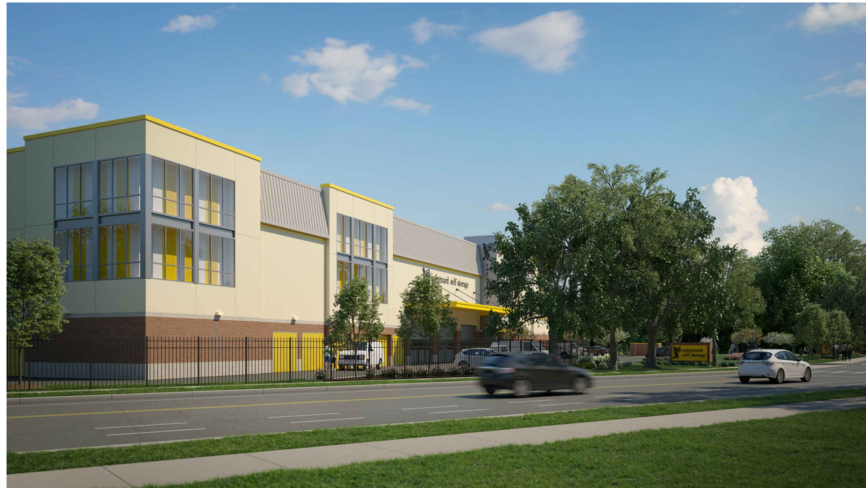
1 LOOKING SOUTHEAST ON HOPE STREET - NEW SCALE: N.T.S.
