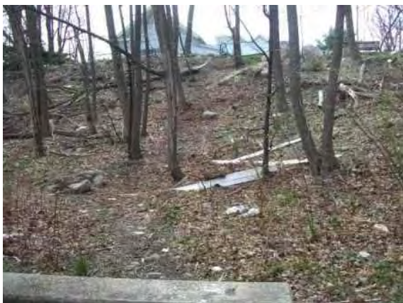
Photo #131: Area of drainage runoff at north parking lot
