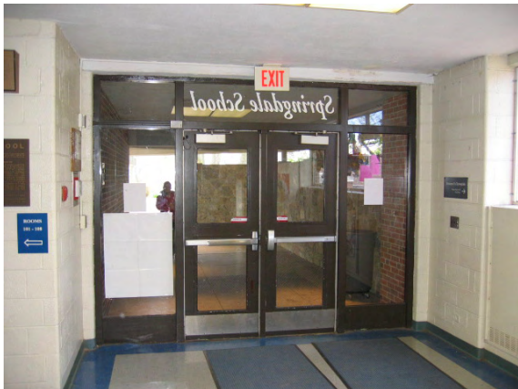
Photo #5: View of the main entrance doors nearest to the office
