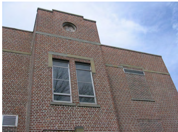
Photo #16: View of the upper front façade
