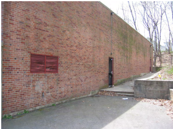
Photo #11: View of the north façade
