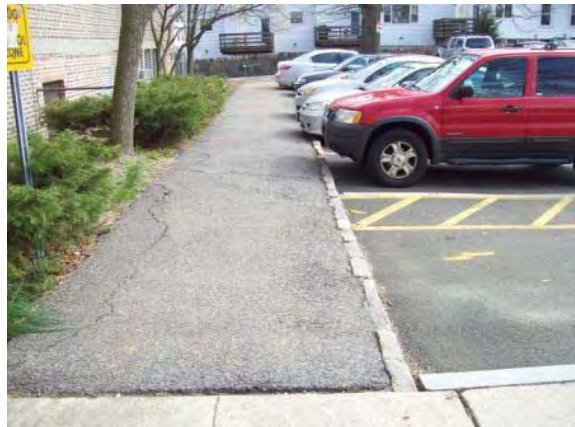
Photo #126: Asphalt sidewalk along front elevation
