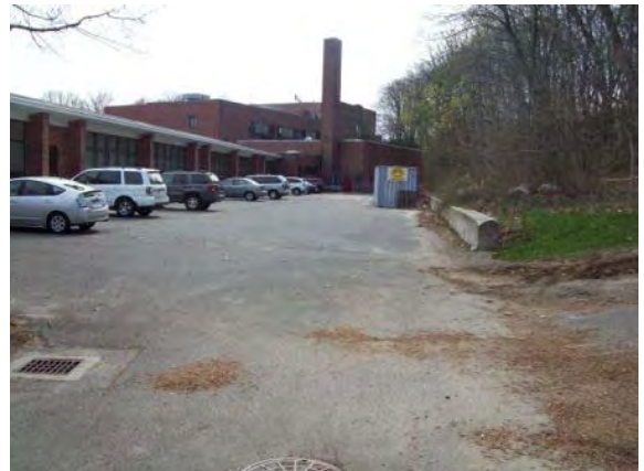
Photo #120: Maintenance parking lot
