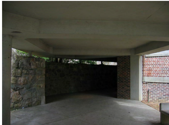
Photo #4: View of the main entrance tunnel
