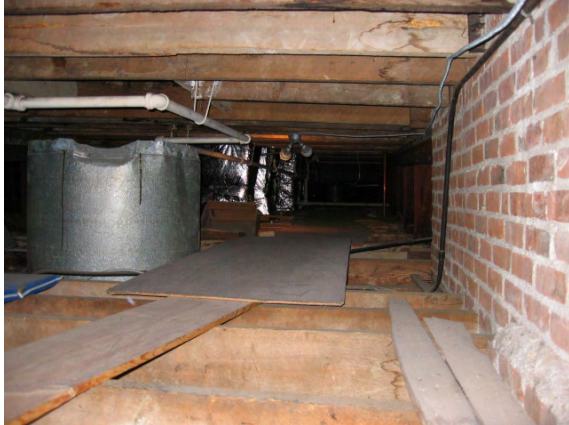
Photo #19: Wood framed attic space beneath the flat primary portion roof
