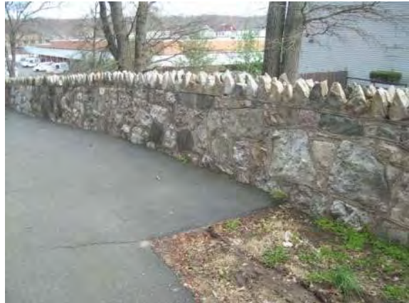
Photo #138: Stone wall at south property line
