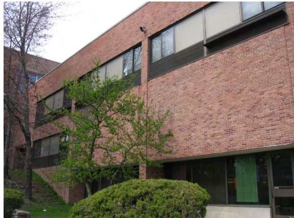
Photo #10: View of the south façade
