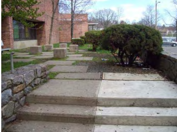
Photo #127: Concrete step and plaza area
