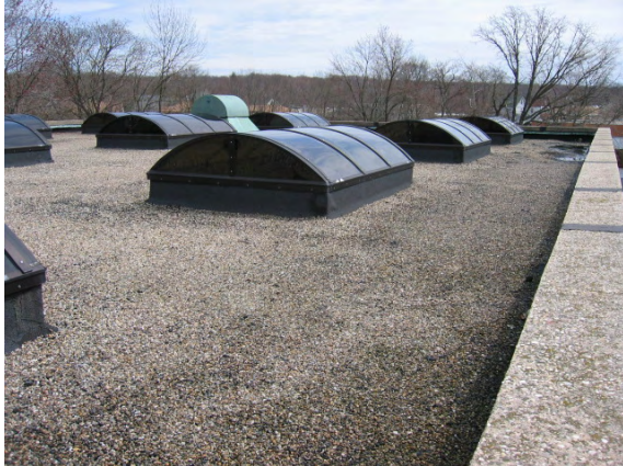
Photo #25: Detail of the gymnasium/ cafeteria roof with barrel type skylights
