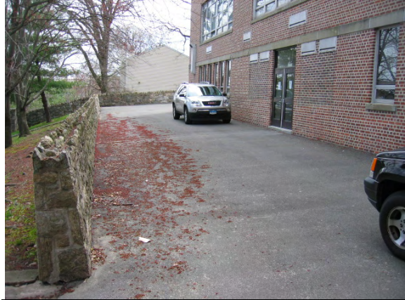
Photo #8: View of the rear façade and asphalt paved driveway
