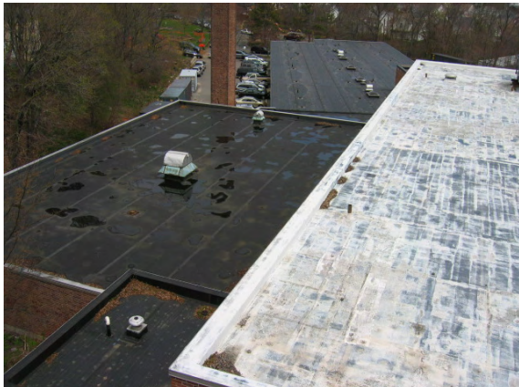
Photo #21: Auditorium and K-1 wing roofs
