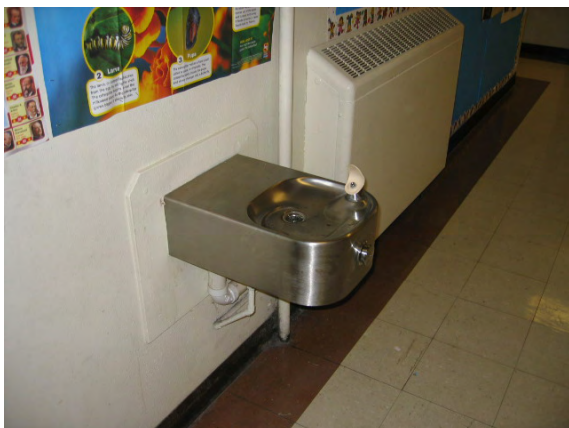
Photo #53: Water fountains project out into the corridor
