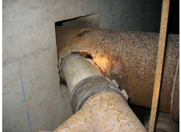
Photo #32: Detail view of a large crack and poorly executed repair at this multi-Y joint
