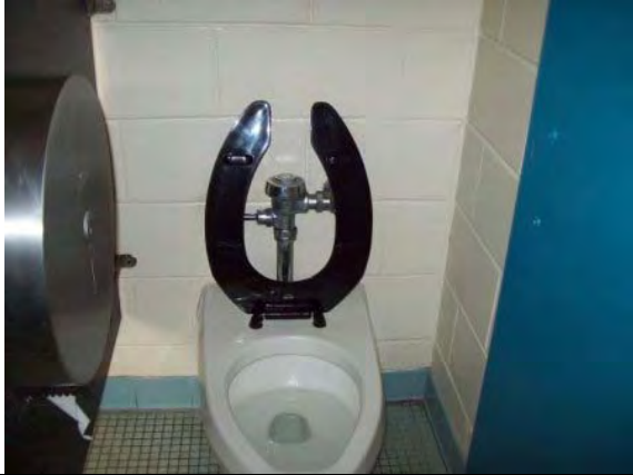
Photo #85: Typical water closet
