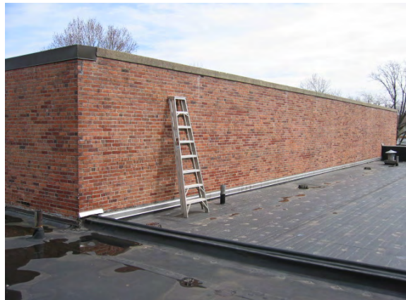
Photo #24: Several of the different roof heights require fixed steel ladders
