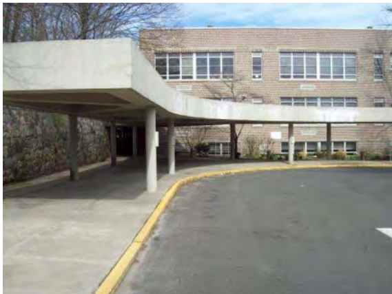
Photo #125: Concrete sidewalks at front of building
