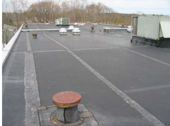
Photo #20: Overview of the main flat, fully adhered EPDM roof system
