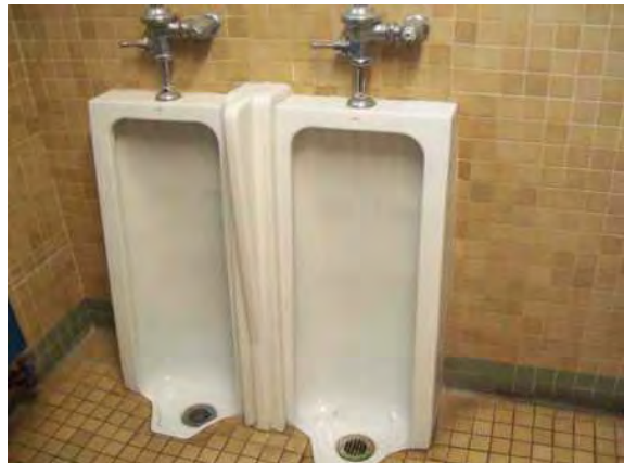
Photo #84: Old floor mounted urinal fixtures
