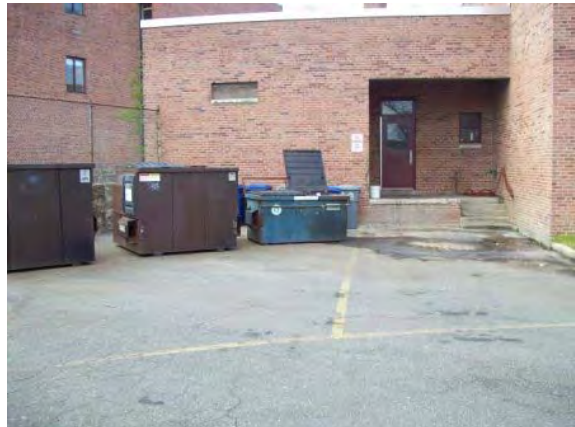
Photo #124: Loading dock
