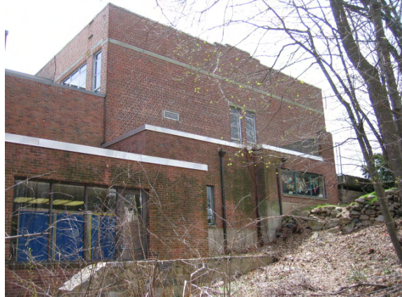
Photo #14: View of the north façade towards the front entrance
