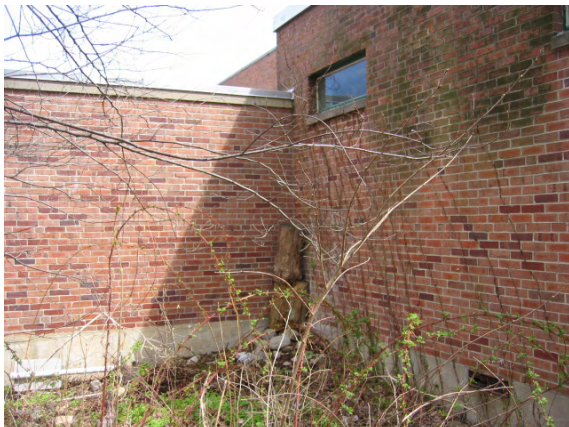
Photo #15: A security fence is needed on top of the auditorium roof
