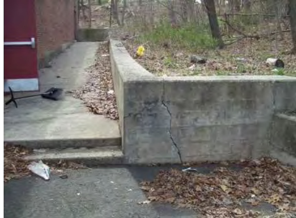
Photo #140: Concrete retaining wall near boiler room
