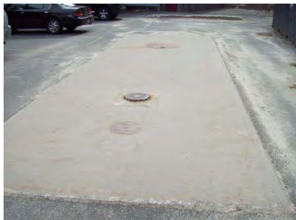
Photo #144: Fuel oil UST location
