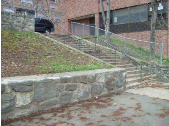
Photo #139: Stone retaining wall along play area
