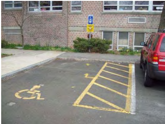
Photo #117: Accessible parking
