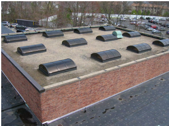
Photo #23: Overview of the gymnasium/cafeteria flat, gravel surfaced built-up roof
