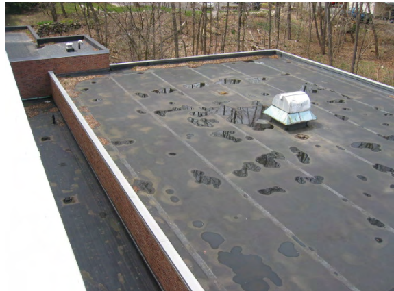
Photo #22: Second view of the auditorium and rear corridor roofs
