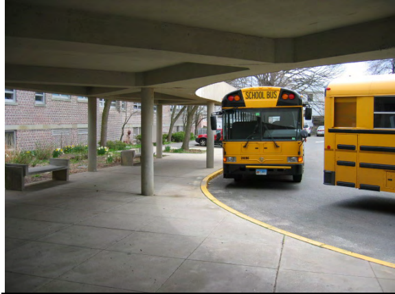
Photo #2: View of the column supported concrete shelter at the bus lane
