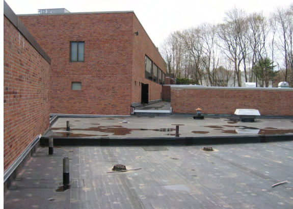
Photo #26: View towards the west of the different EPDM roof systems
