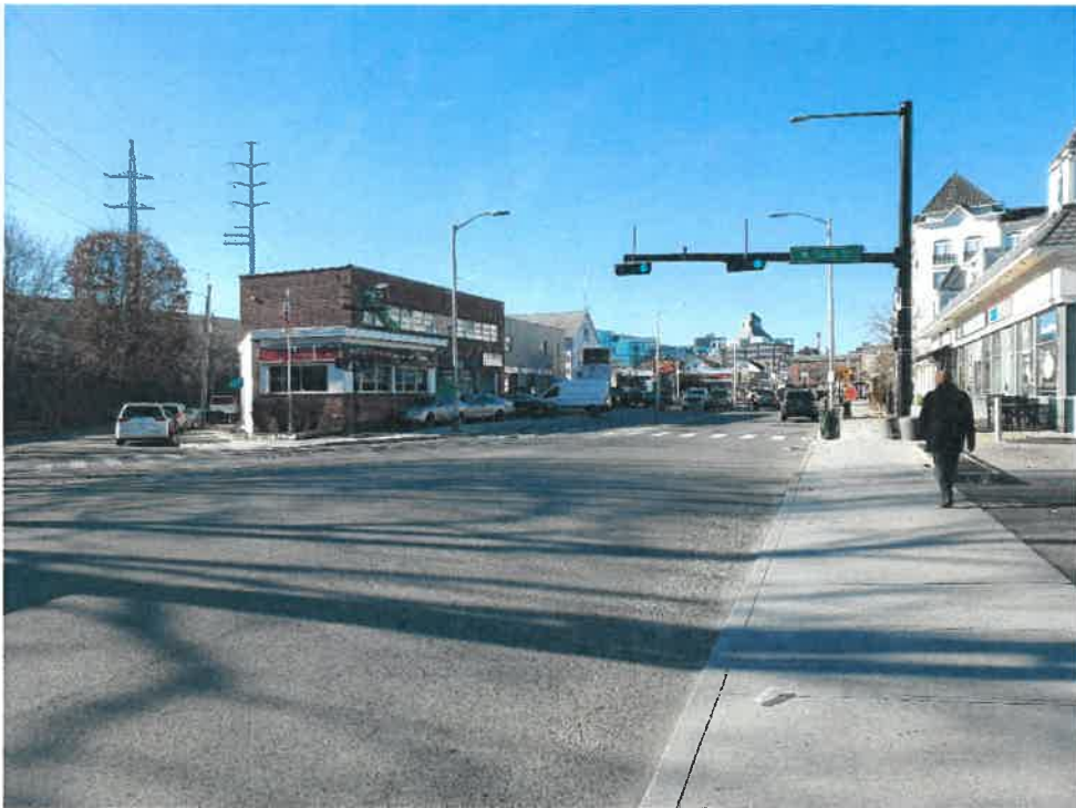
U.S. Route 1 at North State Street Looking West
