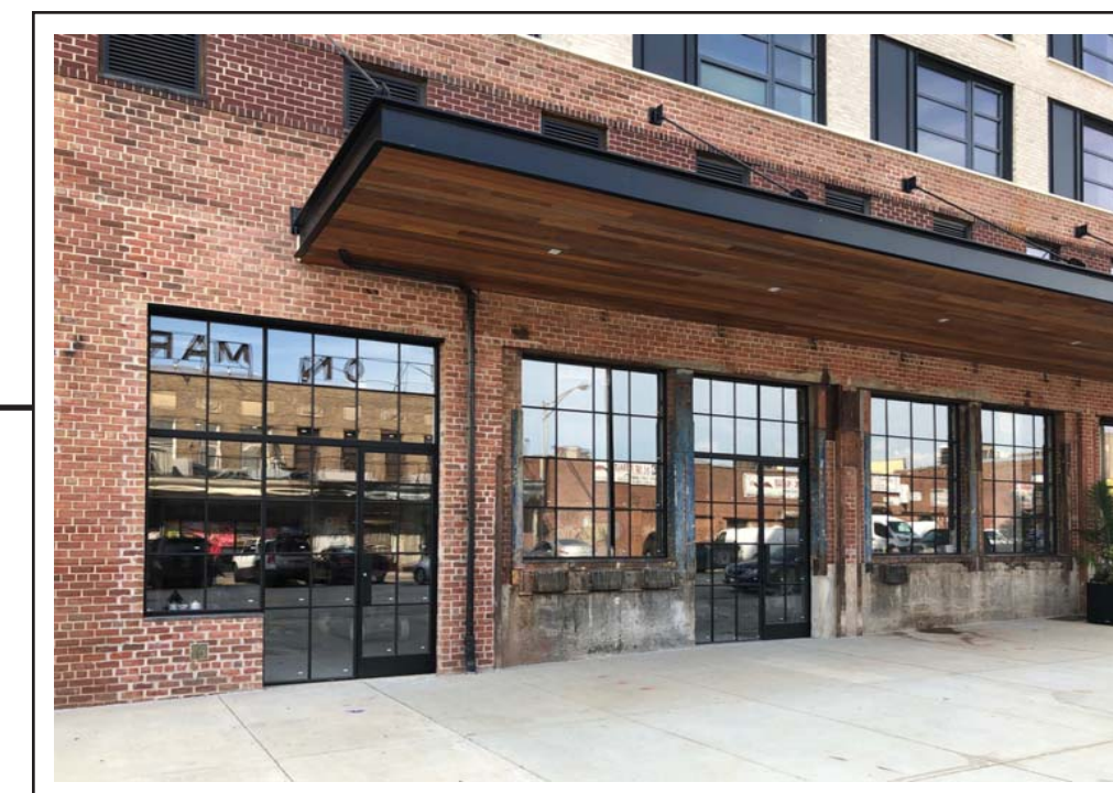
METAL CANOPY & STOREFRONT WINDOWS
