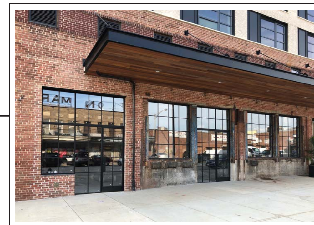
METAL CANOPY & STOREFRONT WINDOWS
