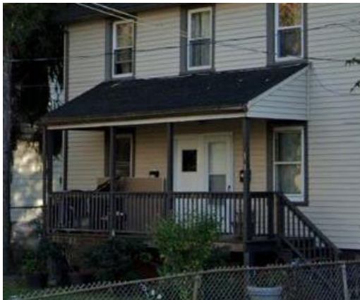
Existing porch (present day)
