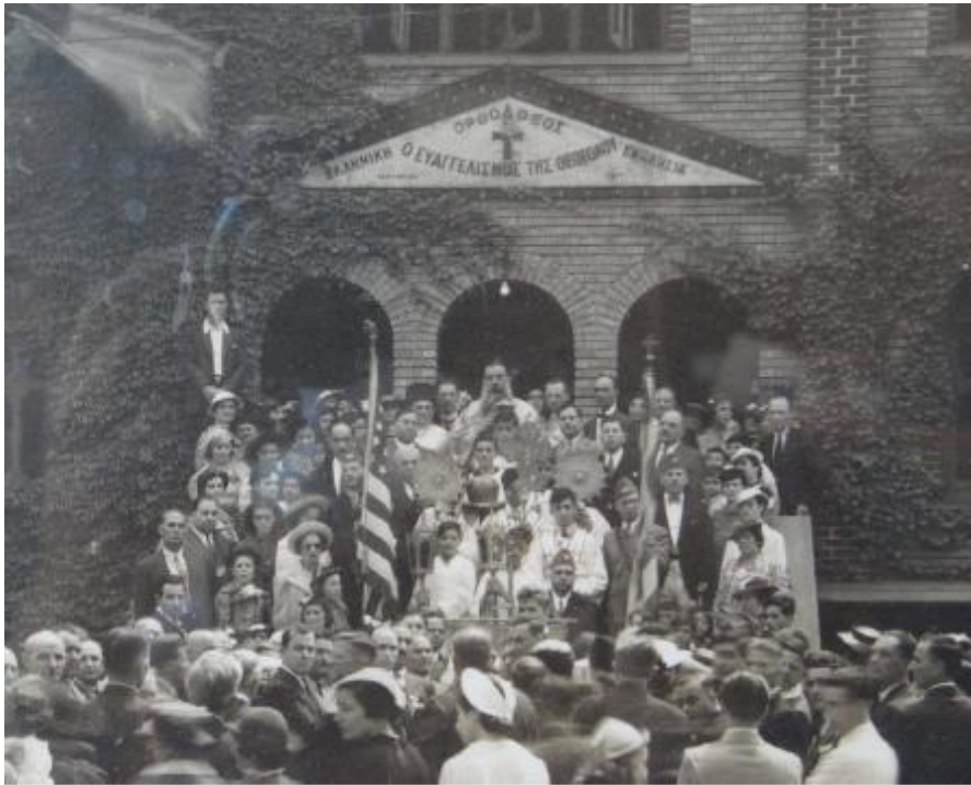
No fixtures on historic building
