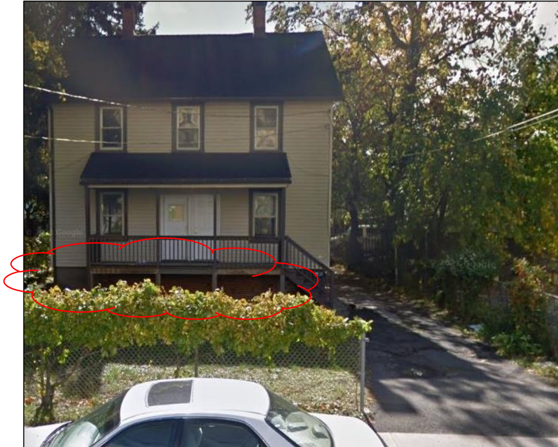
Existing porch (present day)
