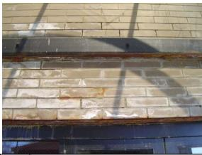
Photo Resulting steel corrosion from failed #118: canopy caulk joints
