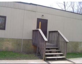
Photo Exit staircase requiring proper handrails #102:
