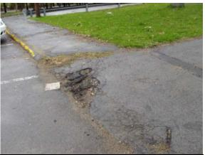
Photo Asphalt sidewalk deterioration at rear of #150: building
