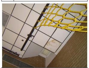
Photo Water intrusion into gymnasium from #87: exterior wall base leaks
