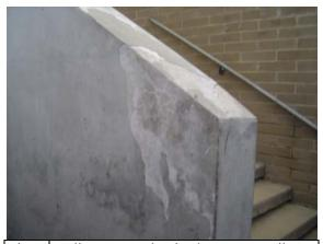
Photo Spalling stucco finish of staircase wall #121: within staircase
