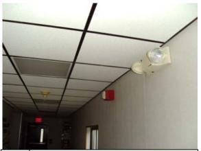
Photo Illuminated exit sign, smoke detector, #226: strobe alarm and emergency lights at modular building
