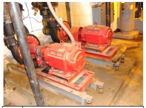
Photo Chilled water circulating pumps #181:
