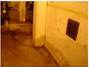
Photo Water intrusion through slab and wall #58: base in boiler room
