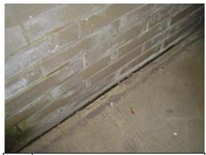
Photo Water damaged brick veneer along #122: landing within staircase
