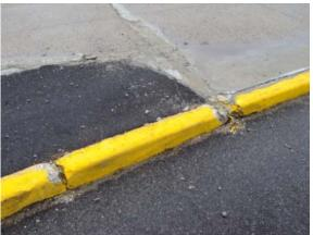
Photo Concrete curbing deterioration at front of #156: building
