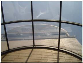
Photo Impact damage on Intra-building walkway #117: canopy plexiglass panels
