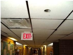
Photo Illuminated exit sign and sprinkler head – #224: note missing escutcheon and cover
