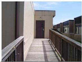
Photo Missing handrails on ADA ramp of #104: modular building
