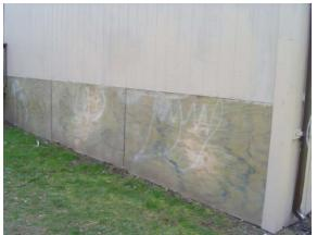
Photo Modular building base panels requiring #103: replacement due to water damage
