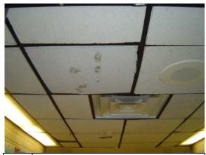
Photo Suspect mold growth on corridor ceiling #68: tiles adjacent to classroom 33
