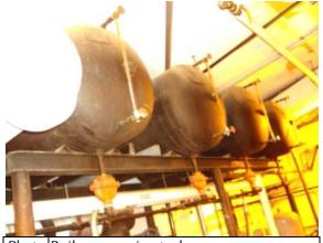
Photo Boiler expansion tanks #179:
