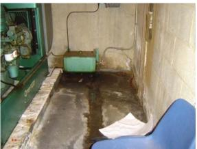
Photo Water intrusion into electrical generator #60: room
