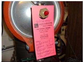
Photo Failed 2<sup>nd</sup> check assembly at fire #218: suppression equipment
