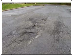
Photo Asphalt deterioration at front parking lot #135:
