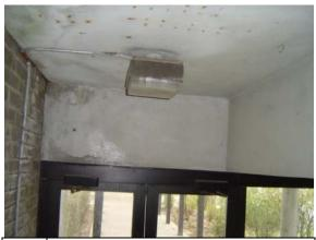
Photo Water damaged finishes in stairwell #123:
