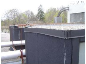
Photo Roof clerestory covers potential source of #53: water intrusion
