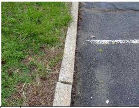
Photo Shifting concrete curbing at front parking #154: lot
