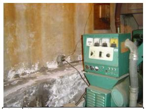
Photo Efflorescence on generator room #61: foundation wall
