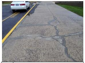
Photo Concrete sidewalk condition at front of the #145: building
