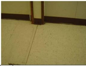
Photo Cracked floor tile in modular building #82:
