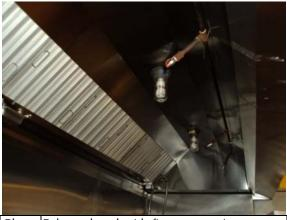
Photo Exhaust hood with fire suppression #221:
