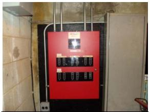
Photo Central fire alarm panel in basement #215: mechanical room
