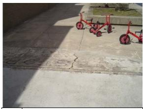
Photo Broken concrete and wall to pavement #92: base allowing for water intrusion
