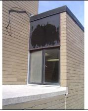
Photo Peeling factory finish of window spandrel #126: panel
