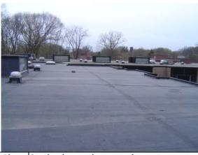
Photo Single-ply membrane roof overview #22:
