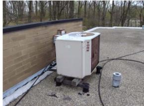
Photo Rooftop condensing unit for office #176:
