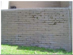
Photo Mildew growth and effervescence on #105: brick veneer along the west elevation
