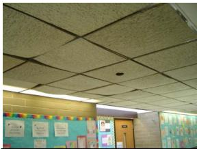
Photo Typical warped ceiling tiles in corridor #67: requiring replacement
