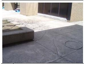
Photo Broken concrete in courtyard and #91: perimeter wall to base water intrusion
