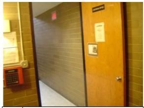
Photo ADA lever handles required on interior #74:
