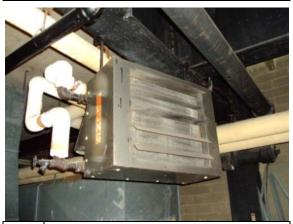
Photo Ceiling-mounted unit heater at mechanical #191: room
