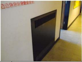
Photo Recessed cabinet radiant unit at corridor #183:
