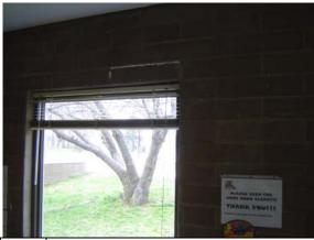
Photo Water intrusion through window of the #76: main office
