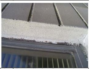
Photo Close-up of brittle caulking around #125: building windows
