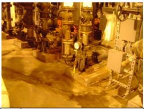
Photo Water intrusion through slab in boiler #57: room
