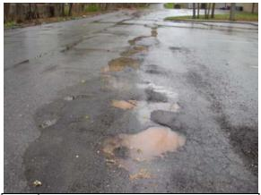
Photo Asphalt deterioration at rear parking and #139: basketball courts
