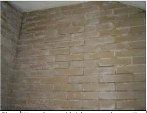
Photo Water damaged brick veneer along ceiling #120: within staircase
