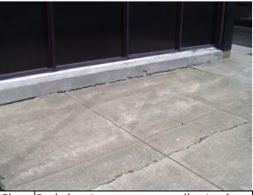
Photo Settled perimeter pavement allowing for #90: water intrusion
