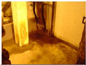
Photo Water intrusion through slab pipe #56: penetrations in boiler room
