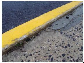
Photo Settled concrete sidewalk – trip hazard at #146: front of building
