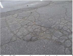
Photo Alligator cracking at asphalt at front #138: parking lot
