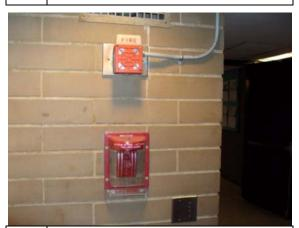
Photo Fire pull station and strobe alarm #225:
