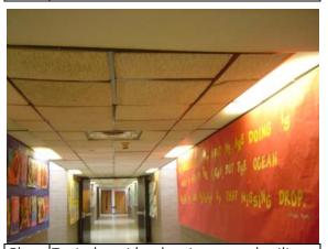
Photo Typical corridor showing warped ceiling #35: tiles requiring replacement
