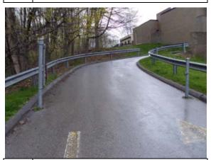
Photo Asphalt curbing along rear service drive #153:
