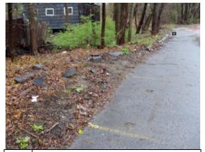
Photo Displaced asphalt curbing at rear of building
