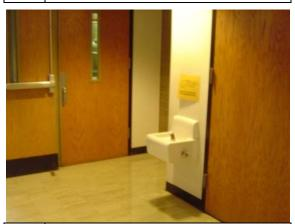
Photo Typical fountain requiring ADA cane #75: detection
