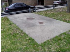
Photo Underground 10,000-gallon fuel oil #178: storage tank at rear of building
