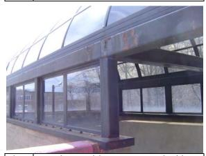
Photo Corroding steel framing on Intra-building #119: walkway canopy
