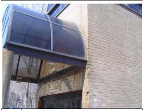
Photo Failed caulk joints on Intra-building #114: walkway canopy and broken veneer
