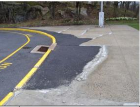
Photo Asphalt overlay on concrete sidewalk at #148: front of building – notice deterioration
