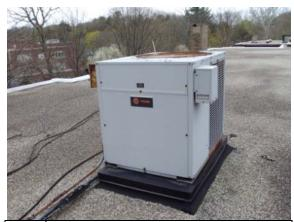
Photo Rooftop condensing unit for computer #175: labs
