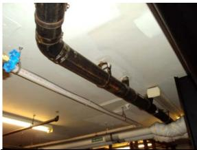
Photo Cast iron plumbing piping #194:
