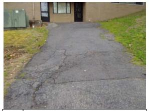
Photo Asphalt sidewalk deterioration at rear of #151: building
