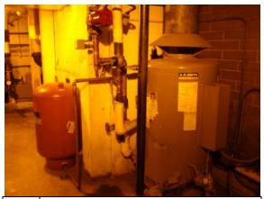
Photo Domestic hot water boiler, circulator and #193: expansion tank
