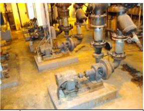
Photo Hot water circulating pumps #180:
