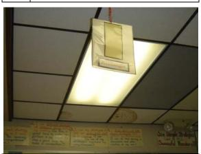
Photo Suspect mold growth on ceiling tile in #63: classroom P4
