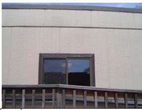
Photo Modular building peeling window frame #106:
