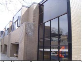
Photo Curtain wall worn and corroding factory #94: finish
