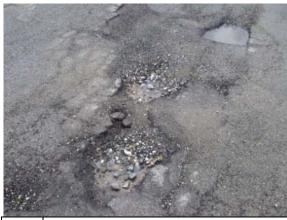
Photo Asphalt deterioration at front parking lot #136:
