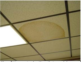
Photo Water stained ceiling tile in modular #66: building
