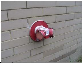
Photo Siamese hose connection at building #220: exterior wall
