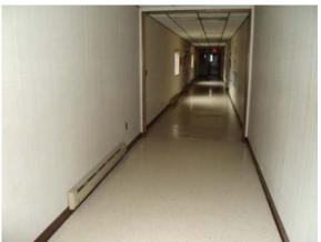
Photo Electric baseboard heaters at modular #192: building corridor
