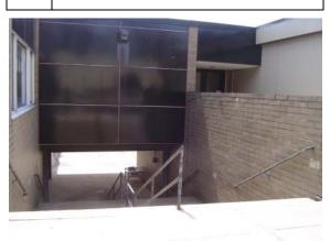
Photo Retaining wall and handrails requiring #99: repairs
