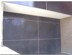
Photo Peeling factory finish of spandrel panel #124:
