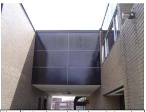
Photo Peeling factory finish of spandrel panel #93:
