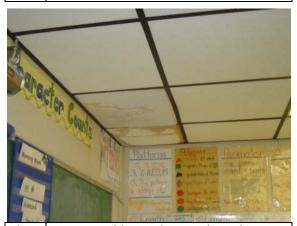
Photo Suspect mold growth on ceiling tile in #65: classroom P4
