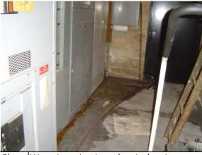
Photo Water intrusion into electrical mains room #59:
