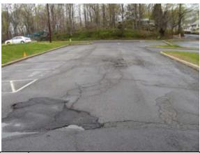
Photo Asphalt deterioration at front parking lot #137:
