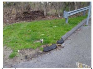
Photo Asphalt curbing deterioration at rear of #158: building
