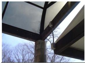
Photo Corroding steel framing on Intra-building #116: walkway canopy
