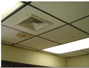
Photo Suspect mold growth on ceiling tile in #64: classroom P3
