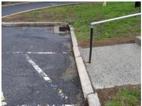
Photo Shifting concrete curbing adjacent to front #155: steps and drain inlet
