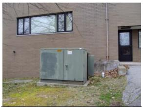
Photo Pad-mounted transformer at rear of #203: building
