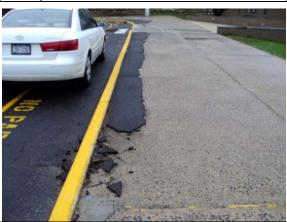
Photo Asphalt overlay on concrete sidewalk at #147: front of building – deterioration at asphalt
