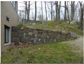
Photo Stone masonry retaining wall at rear #161: elevation
