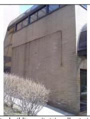
Photo Intra-building exit stairwell exterior wall #111: requiring pointing
