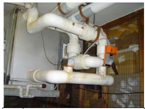
Photo Suspect mold growth on air handling pipe #62: insulation
