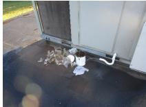
We did not find any items in need of repair on the lower roof level. We did however find garbage and debris by a unit. These need to be removed before they can blow around and cause damage. Servicemen working on the roofs should be asked to remove their garbage. These should not be left on the roof.
