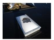
There is a skylight with a broken outer dome present on the roof. The skylight domes should be replaced before too much water can collect inside and work its way in the skylight frame and building.
