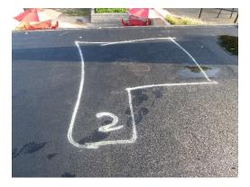
As discussed above, wet area # 2 is the only found area marked on the roof from the moisture scan. It appears the wetness came from holes. There are a few patches in the roof in this area.
