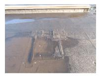
Patches in the roof should be closely examined, especially if they fall within ponding water, to make sure that the laps are tight and not starting to peel. If any looseness is suspected, the laps should be overlaid with PS flashing as a precaution.
