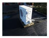
A slip sheet of membrane should be placed between the sleepers for this unit and the roof membrane. The separation sheet is important to prevent rubbing of the membrane by the sleepers. It is also a requirement of all roof manufacturers.
