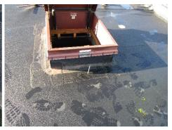
We found a few holes in the roof membrane during our inspection. These occurred in the field of the roof, at the perimeter edge and at curbs. The entire field of the roof, curbs and perimeter edge must be checked, and any holes or damage repaired before more water enters the roof system.
