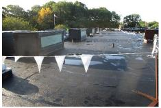
The remaining EPDM roof is in very good shape and only needs a few minor repairs. The roof was flagged off during our inspection because the old BUR roofs on top of the raised light penthouses were being reroofed.
