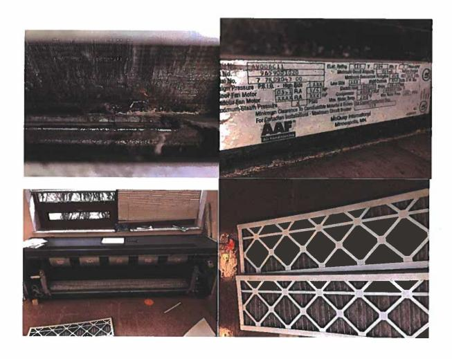
Room A102 UV #11: Inspected UV and Tested Operation
