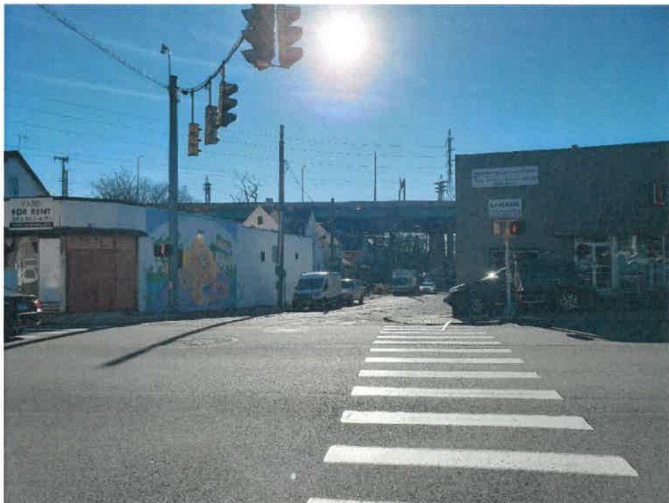
Lafayette Street at U.S. Route 1 Looking South
