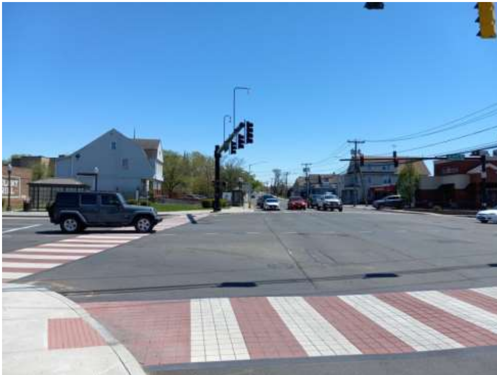
Looking southeast along Elm Street
