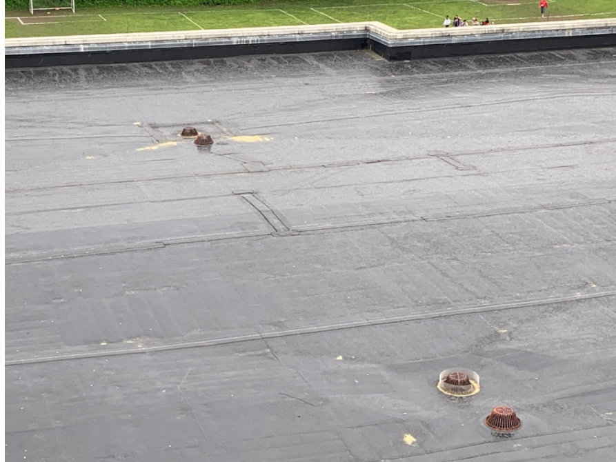
Dry area of roofing
