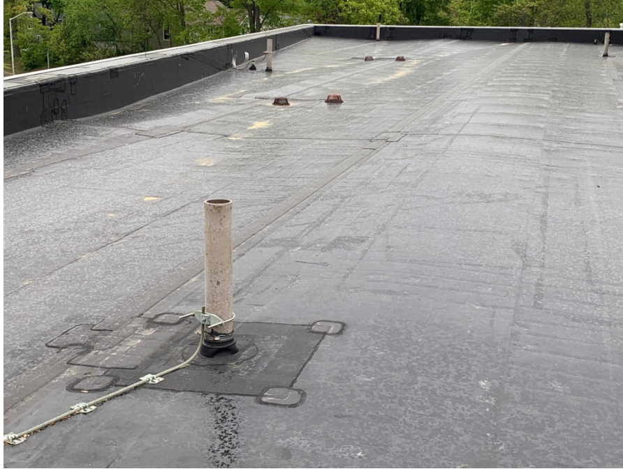
Dry area of roofing
