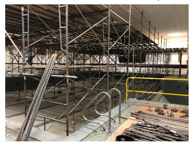
Pool drained and scaffolding erected for ceiling tile replacement, grand stand lighting replacement and installation of new returned air ductwork .
