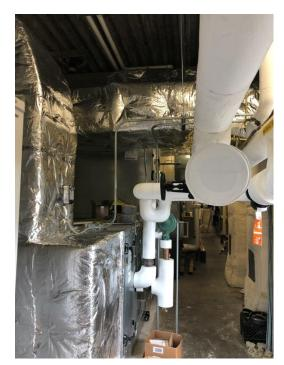
Installed new pool and café air handling units, piping and duct insulation. Pool air handler equipped with de-humidifier.
