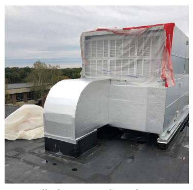
Installed new pool outdoor air energy recovery unit to temper outside air for energy savings required by energy code
