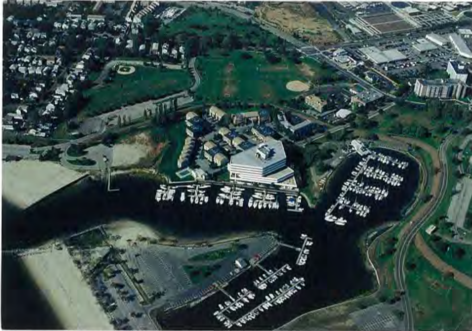
Figure 2-27: Water-dependent facilities in the Cummings Park lagoon include, clockwise from top: Seaview marina; Halloween Yacht Club; and Cummings marina.
