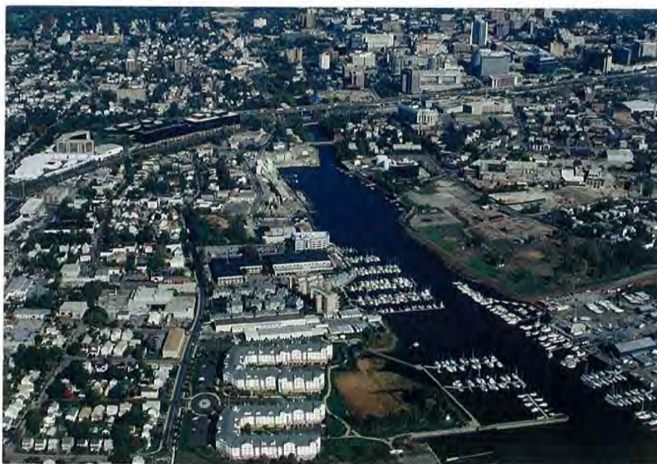
Figure 2-14: Looking upstream on the west branch toward the head of navigation at the Pulaski Street bridge.
