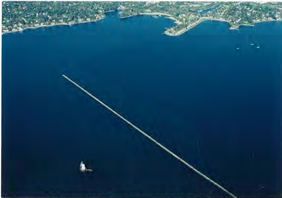
Figure 2-20: West breakwater and Stamford lighthouse in the outer harbor. Peck Point at top of photo.
