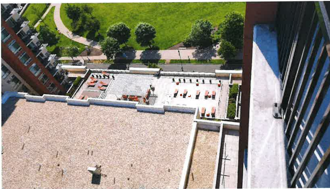
Figure 14- Terrace at East Elevation
