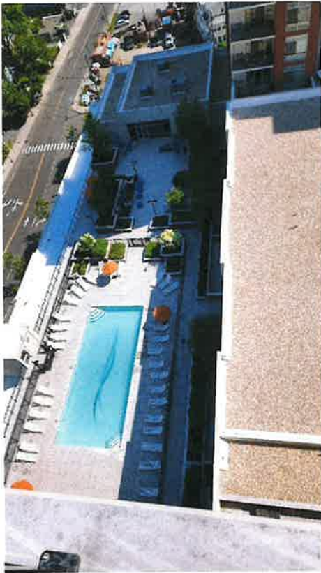
Figure 13- Terrace at West Elevation
