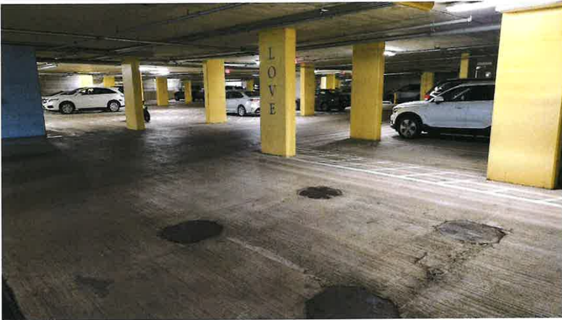
Figure 5- Typical Lower Level of Garage
