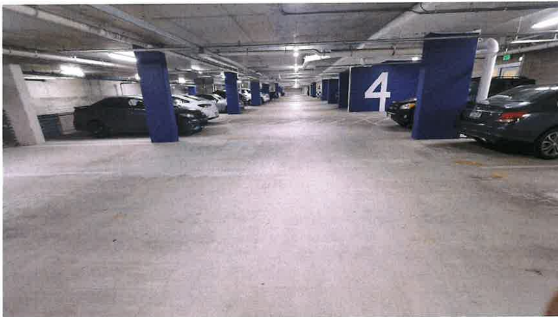
Figure 12-Garage 4 th Floor Level Overall
