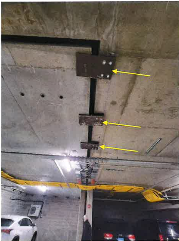
Figure 6- Plates Installed under Expansion Joint
