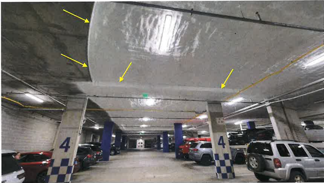
Figure 13- Steps in Slab Beneath Terrace
