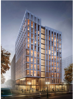
MEDIUM-HIGH FRAMEWORK BUILDING PORTLAND, OREGON
