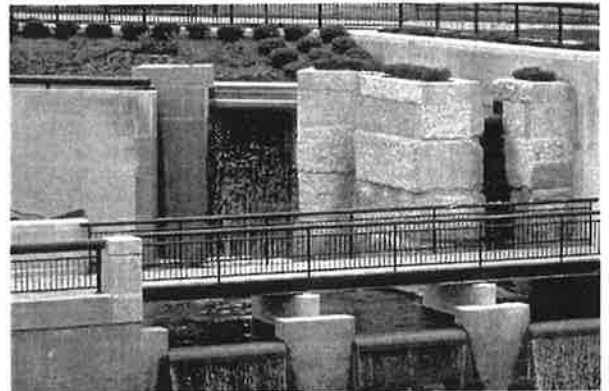
Fig. 48 Example of a dam with pedestrian walkway above it
