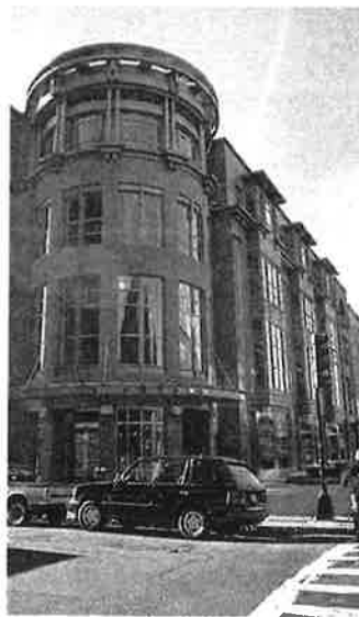
Fig. 15 Tower element pushed out to the property line
