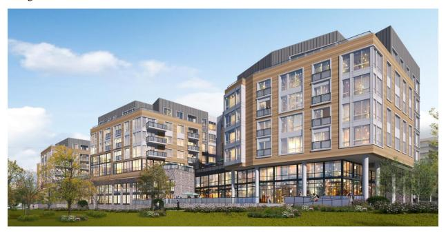
**View of Block B along Mill River** - The proposed development meets the guidelines by providing a clearly defined base, mid-section and top. The punched windows, balconies and setbacks provide relief to the façade. Change in material and framing around the windows help break the building elevation into small portions. Amenity areas are showcased using large glazed windows. Corners are accented using wraparound windows.
