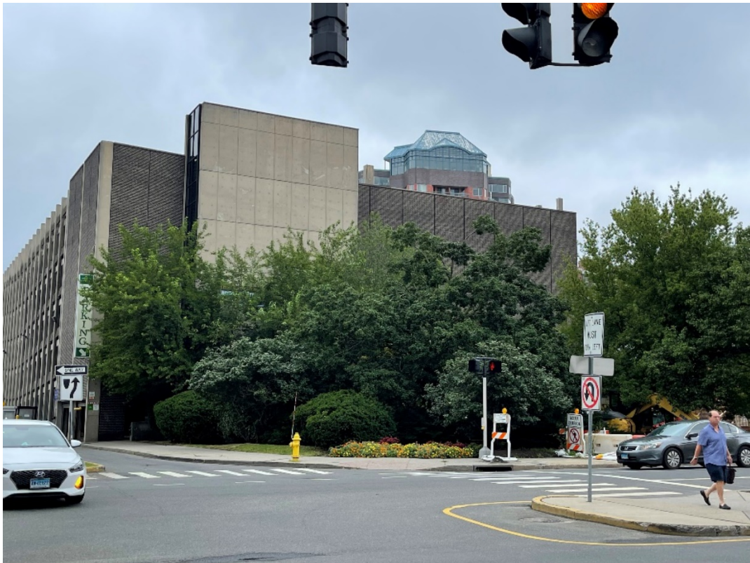
View of 136 Broad Street from other side of Broad Street
