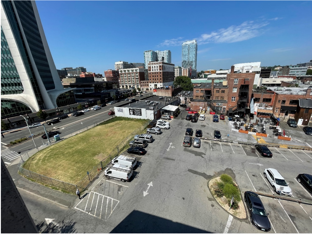
Aerial view of 128 Broad Street and Bedford Street Lot from top of Bedford Street Garage
