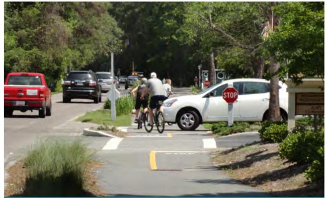
Trails are substantially different from sidepaths. Sidepaths are aligned along a roadway, typically within the roadway right-of-way, and often require users to frequently cross intersections, decreasing safety.
