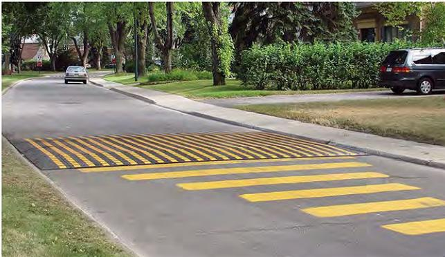
Figure 5 - Moveable rubber speed hump. Photo credit: trafficlogix.com
