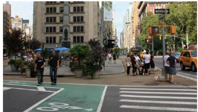
Figure 6 - Temporary bump-out in New York City consisting of paint and aggregate epoxied to existing street pavement. Photo credit: Dave Sousa
