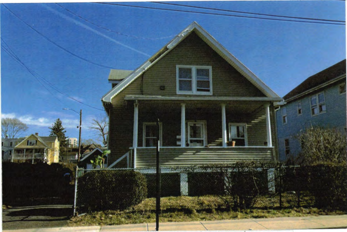
Photograph 1 Facade (South Elevation)
