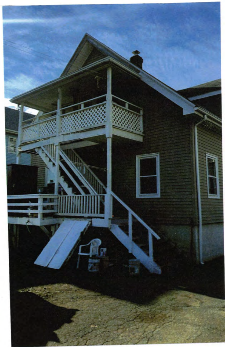
Photograph 8, Rear (North) Elevation
