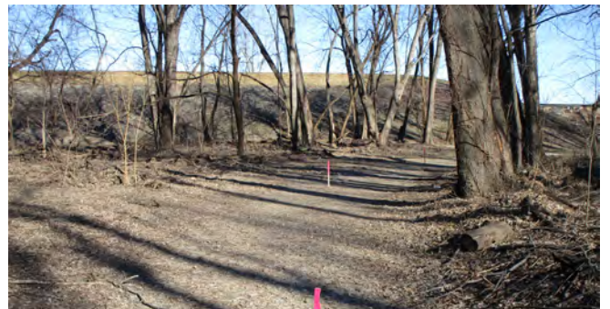
Large Project Area - The Riverwalk North Extension project extends along the Connecticut River from the Greater Hartford Jaycees Community Boathouse northerly for approximately 2.5 miles towards Windsor.
