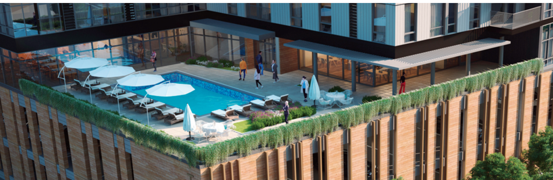
4th Floor Roof Deck - Aerial View
