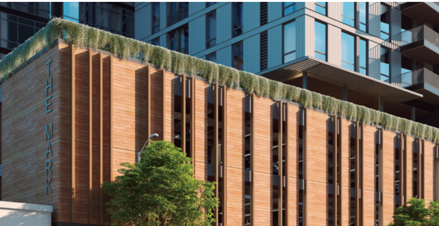
4th Floor Roof Deck - Street View
