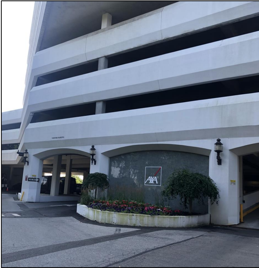
Photo 1: Ground floor view looking southeast from Seaview Avenue.
