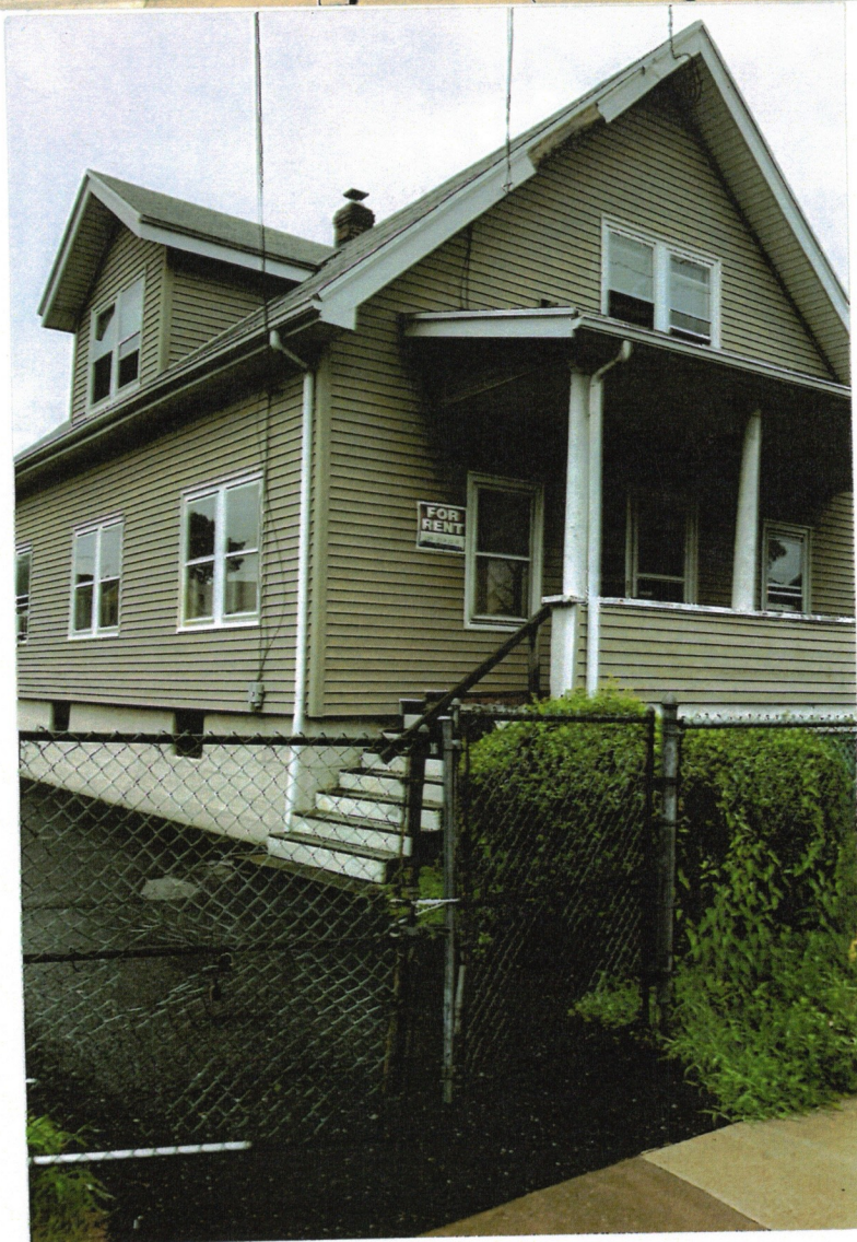
Photograph 2 Facade & West Elevation
