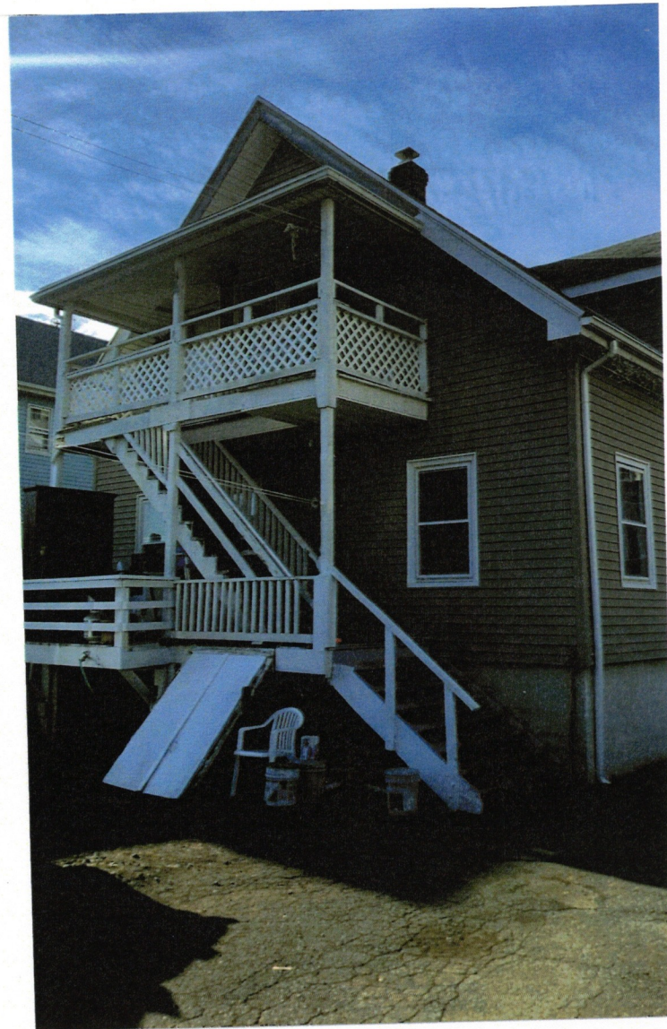
Photograph 8, Rear (North) Elevation
