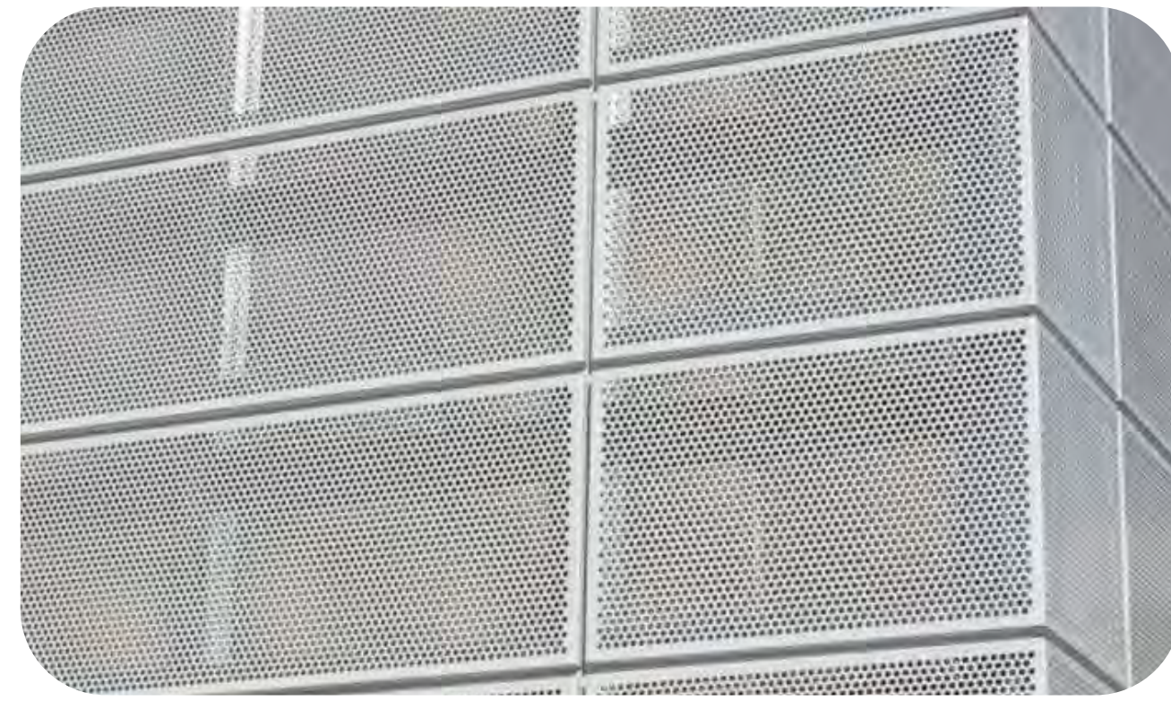
② Perforated metal panel screen / metal screen
