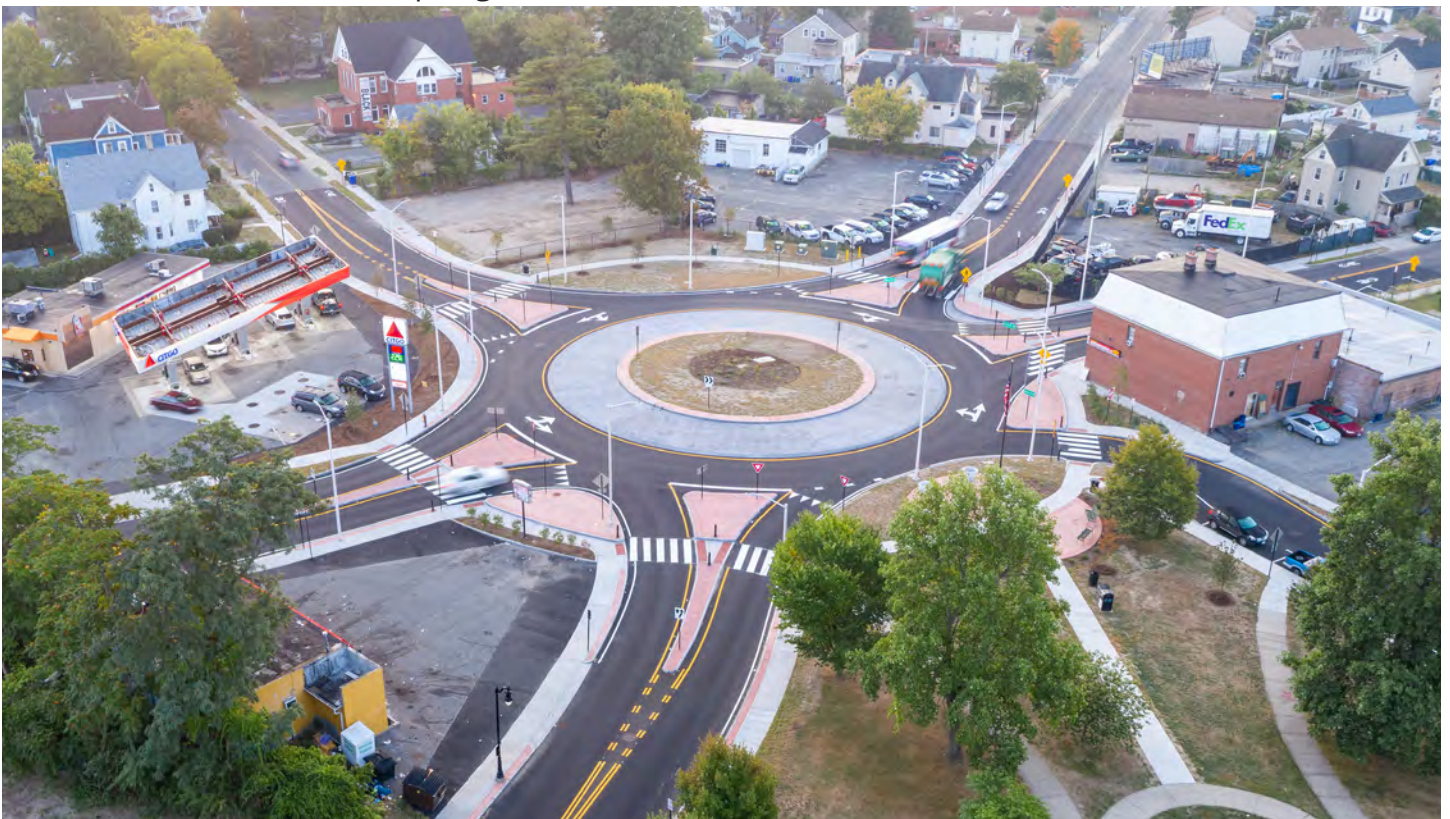
Six Corners Roundabout – Springfield, MA
