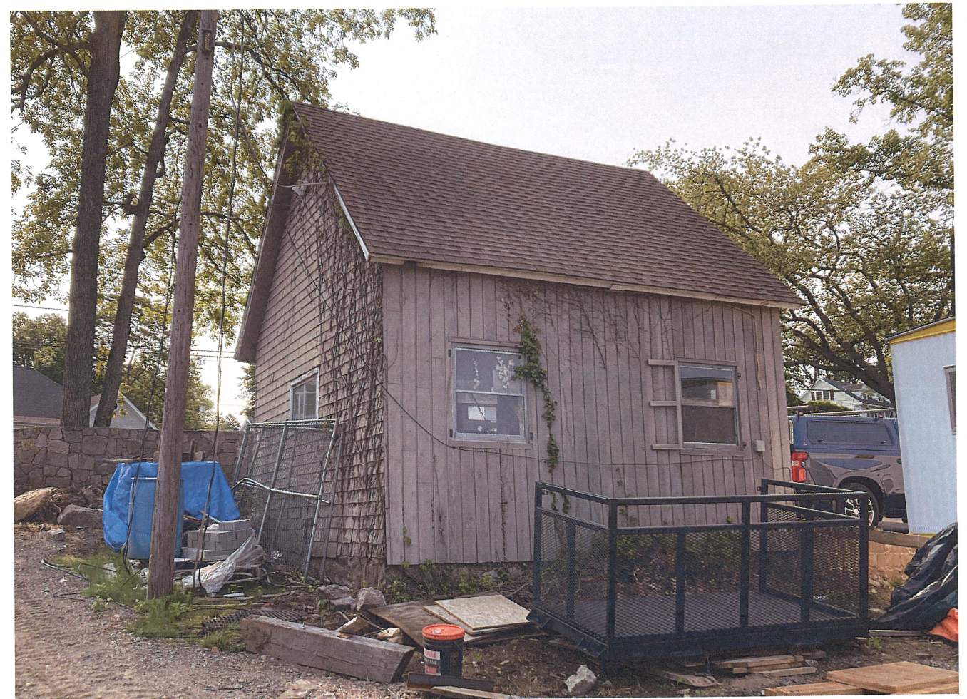
EXISTING BUILDING - VIEW LOOKING EAST
