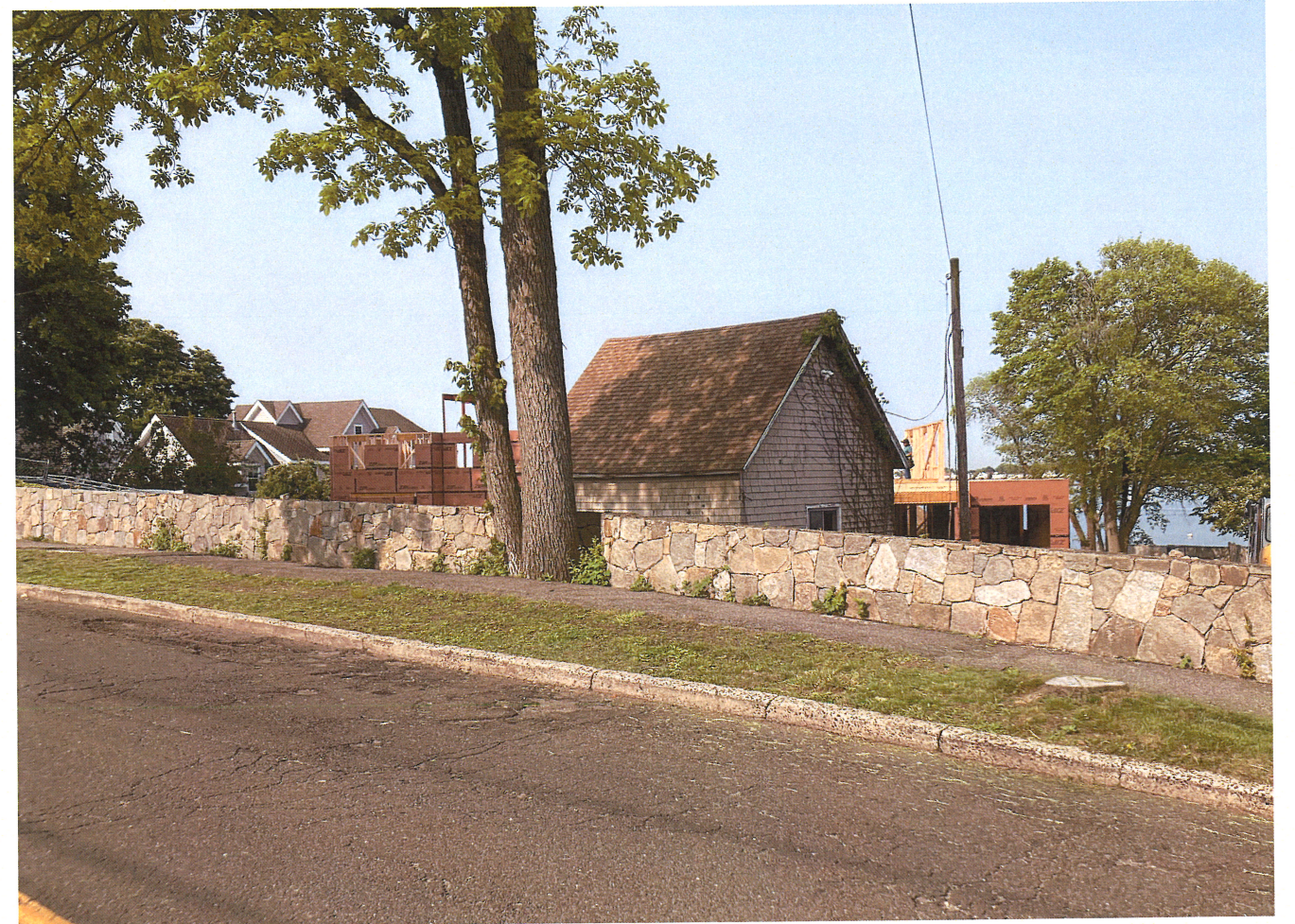
EXISTING BUILDING FROM STREET - VIEW LOOKING SOUTHWEST
