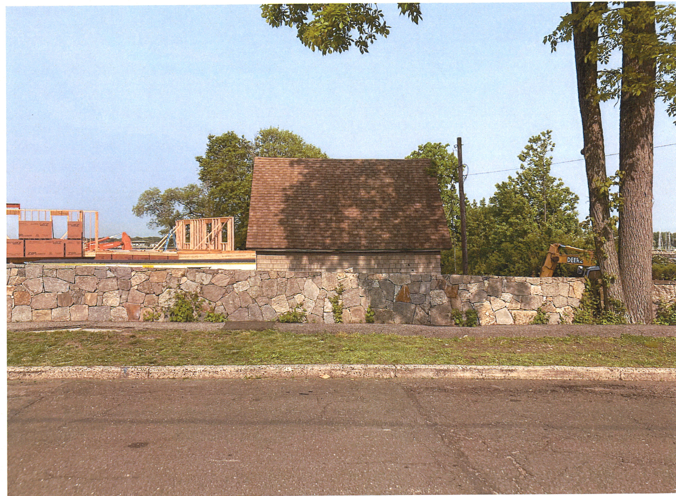
EXISTING BUILDING FROM THE STREET - VIEW LOOKING WEST
