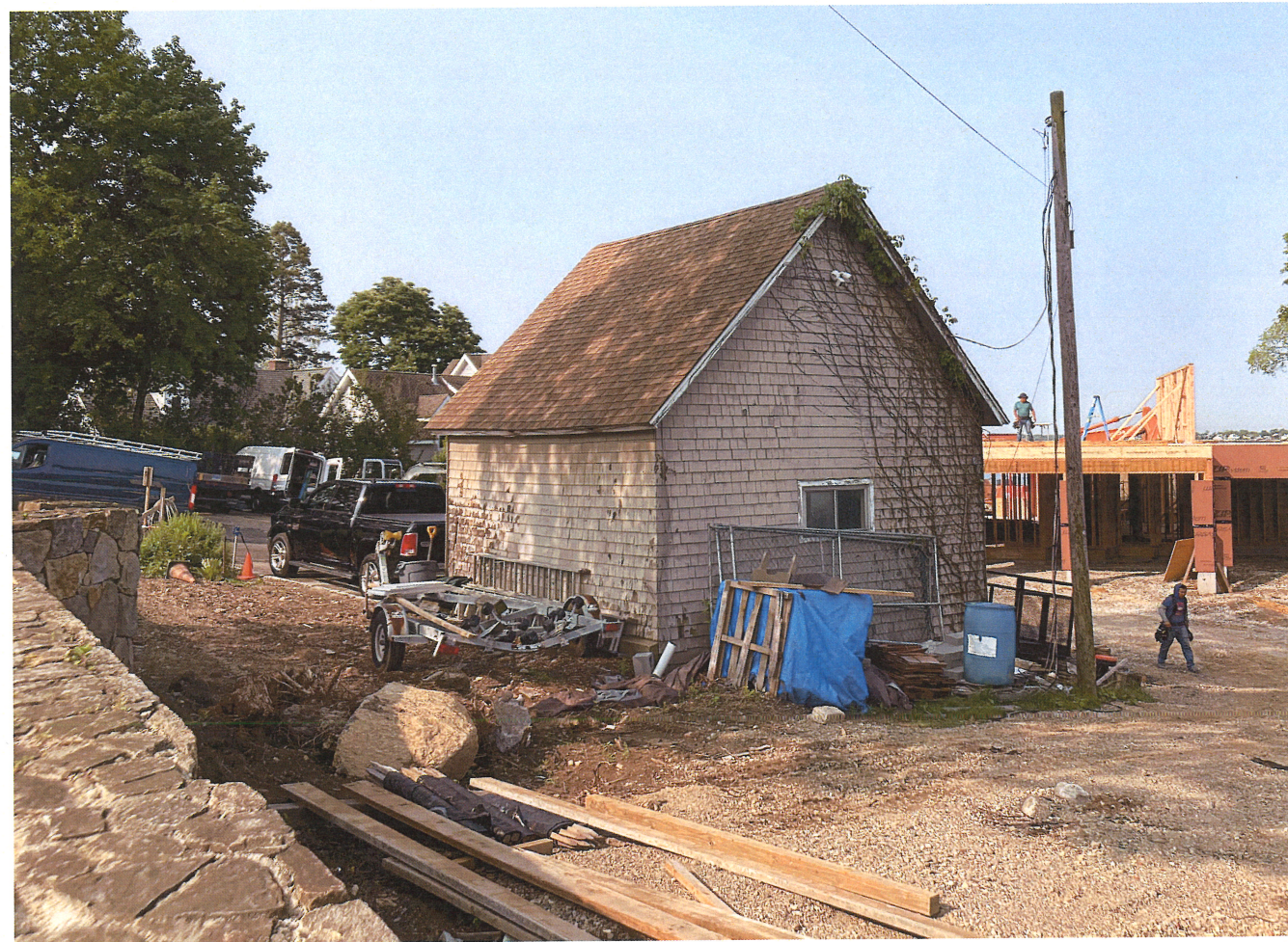
EXISTING BUILDING - VIEW LOOKING SOUTHWEST
