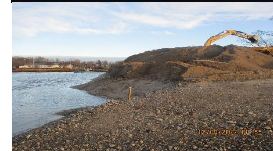
Dredging of Cove
