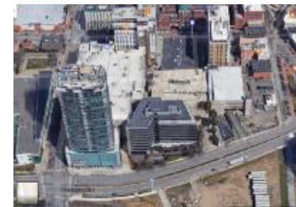
WASHINGTON BLVD SAFETY
