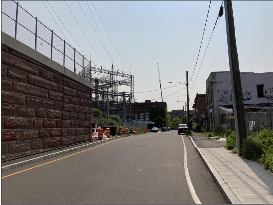
Looking east along Manhattan Street
