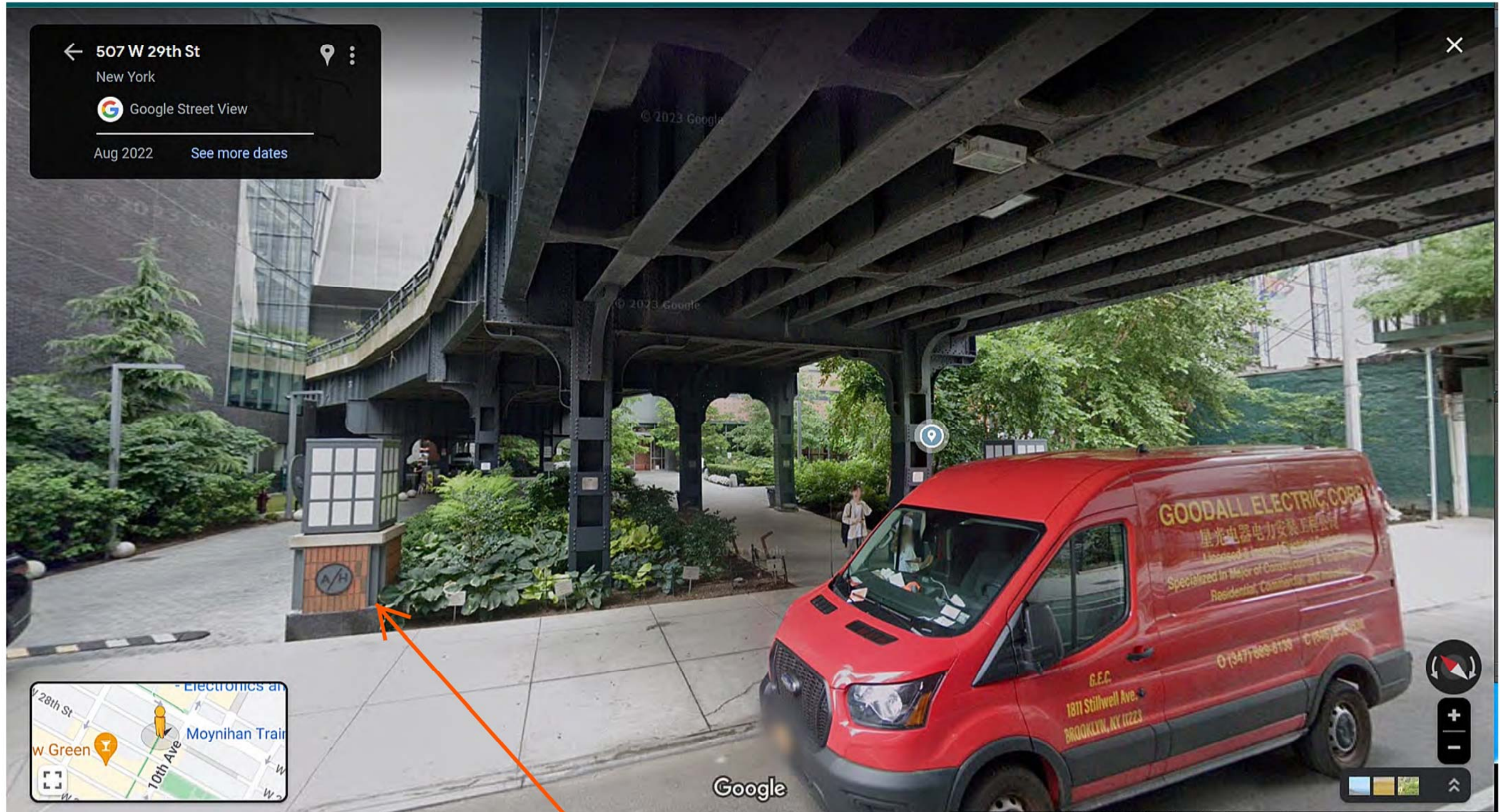
Public area under transportation overpass Bollard/Landscaping lighting elements
