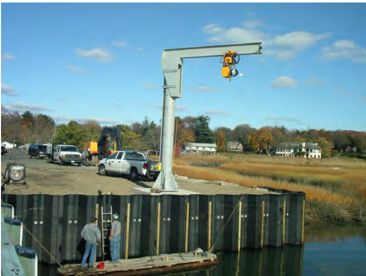
YACHT CLUB DRY-SAIL FACILITY AFTER RACE IMPROVEMENTS
