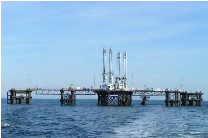
Offshore Unloading Platform
