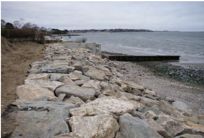
SHORELINE STABILIZATION STRUCTURE
