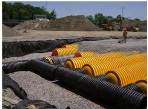
Green infrastructure: storm water infiltrators
