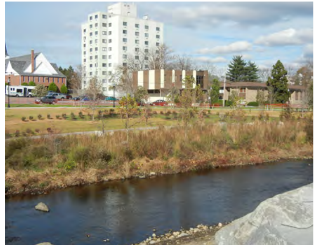
All photos are during the construction of the site
