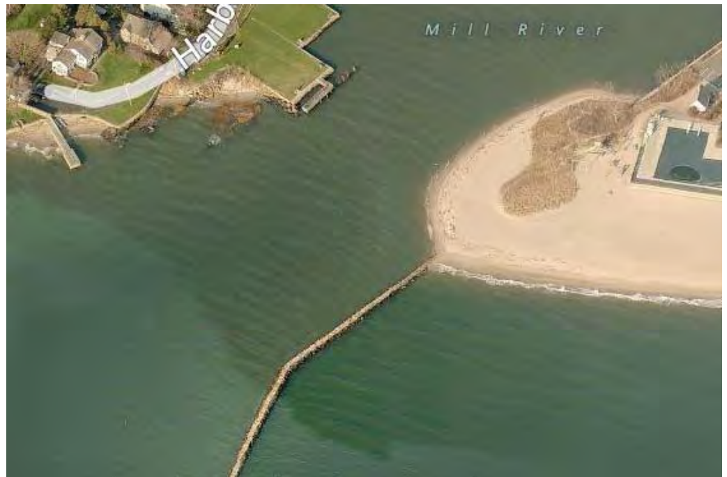
Aerial Photograph of Shoal Area
