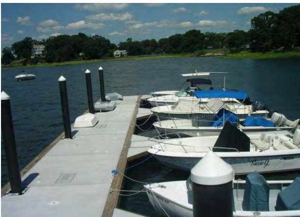
MARINA FLOAT AND ANCHOR PILE IMPROVEMENTS
