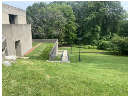
Significant grade difference exists throughout the site
