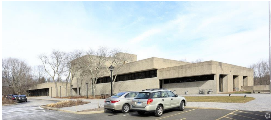
Existing office building (Former C-E/Hyperion)
