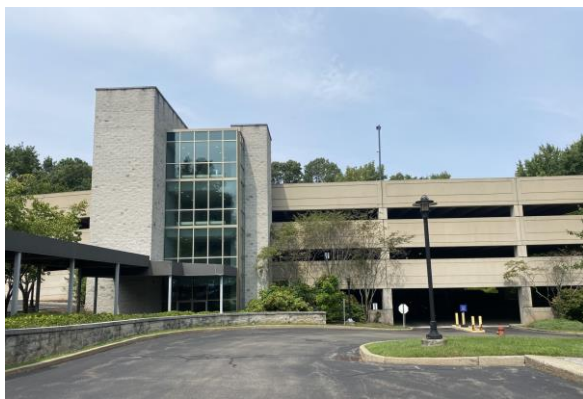
Existing parking garage
