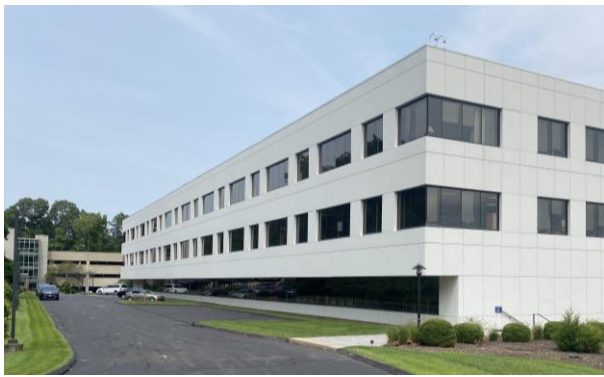
Existing office building (Former Oracle)
