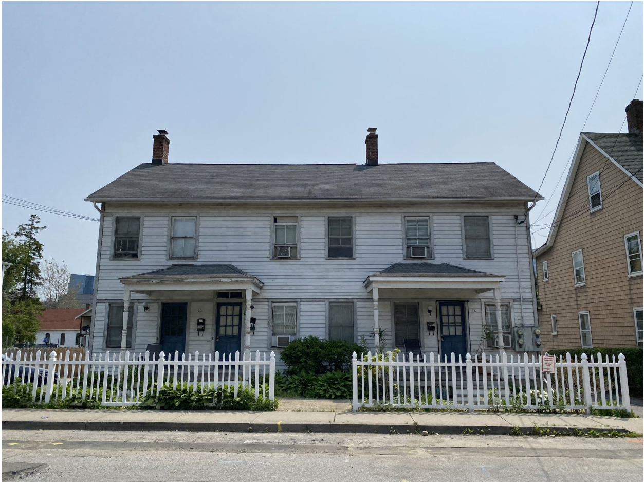
Fig. 1: Current photo of 18 Taylor Street in Stamford Connecticut
