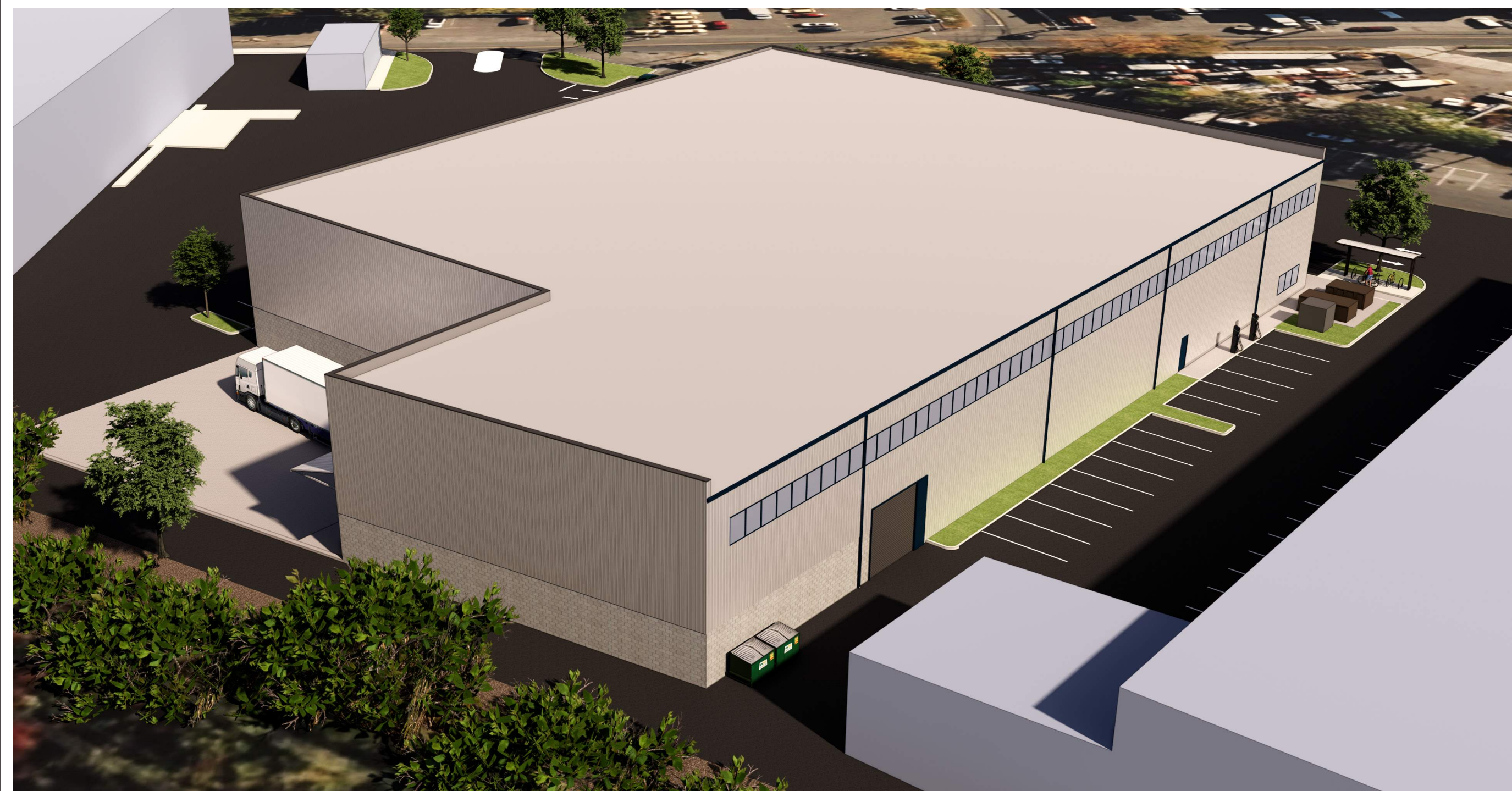
BUILDING B - SOUTHWEST AERIAL VIEW
