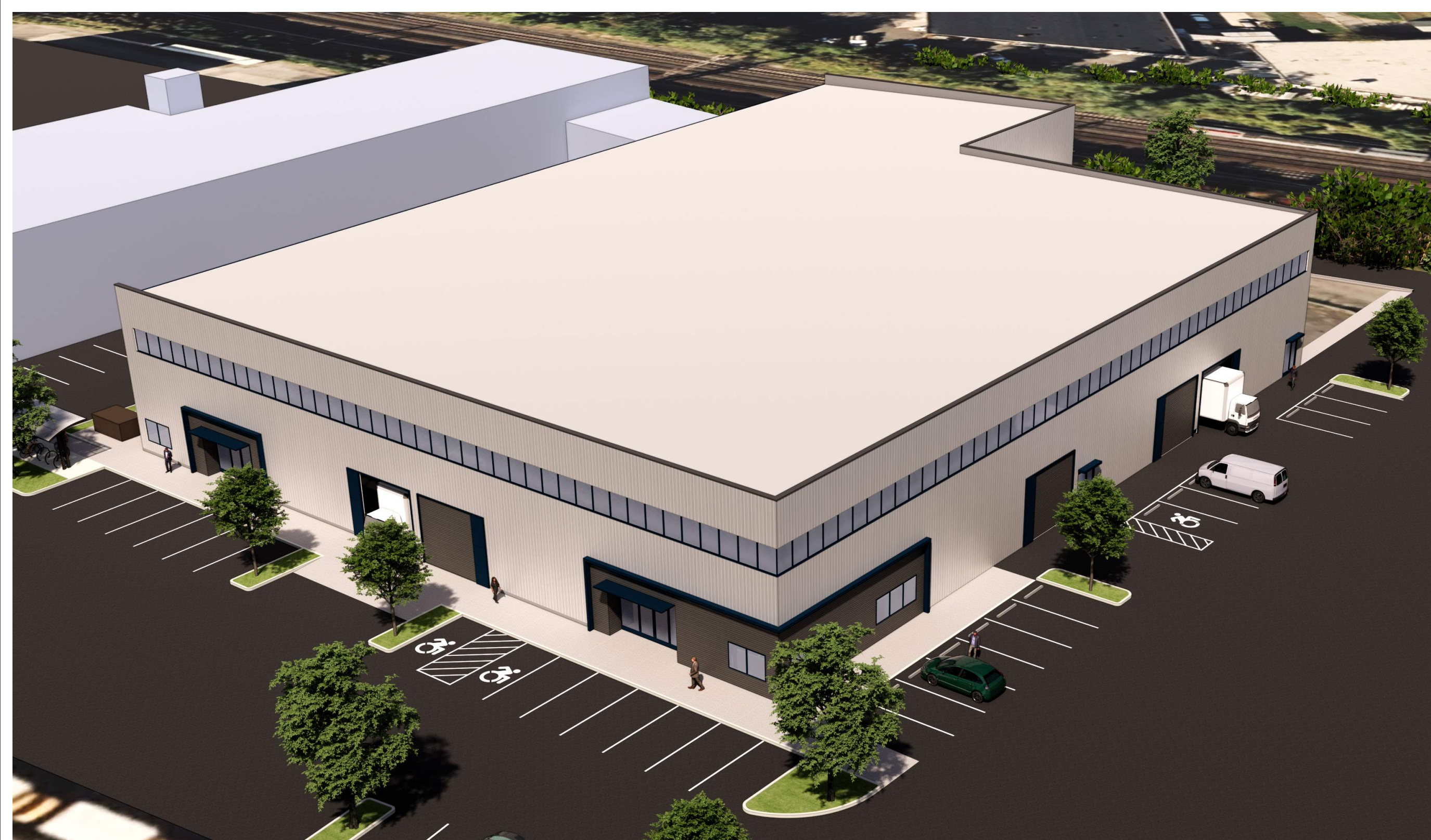
BUILDING B - NORTHEAST AERIAL VIEW
