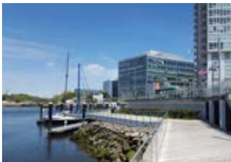
Stamford, CT Permitting modifications to the hurricane barrier.
