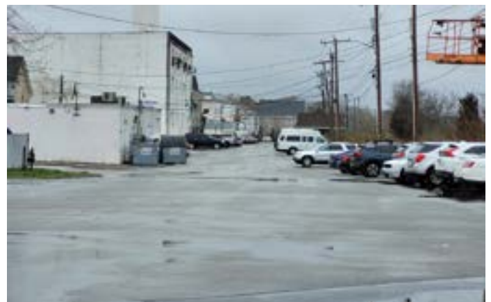
Existing conditions along Merchant's Way between MBTA Cape Flyer rail tracks and the backside of commercial buildings.
