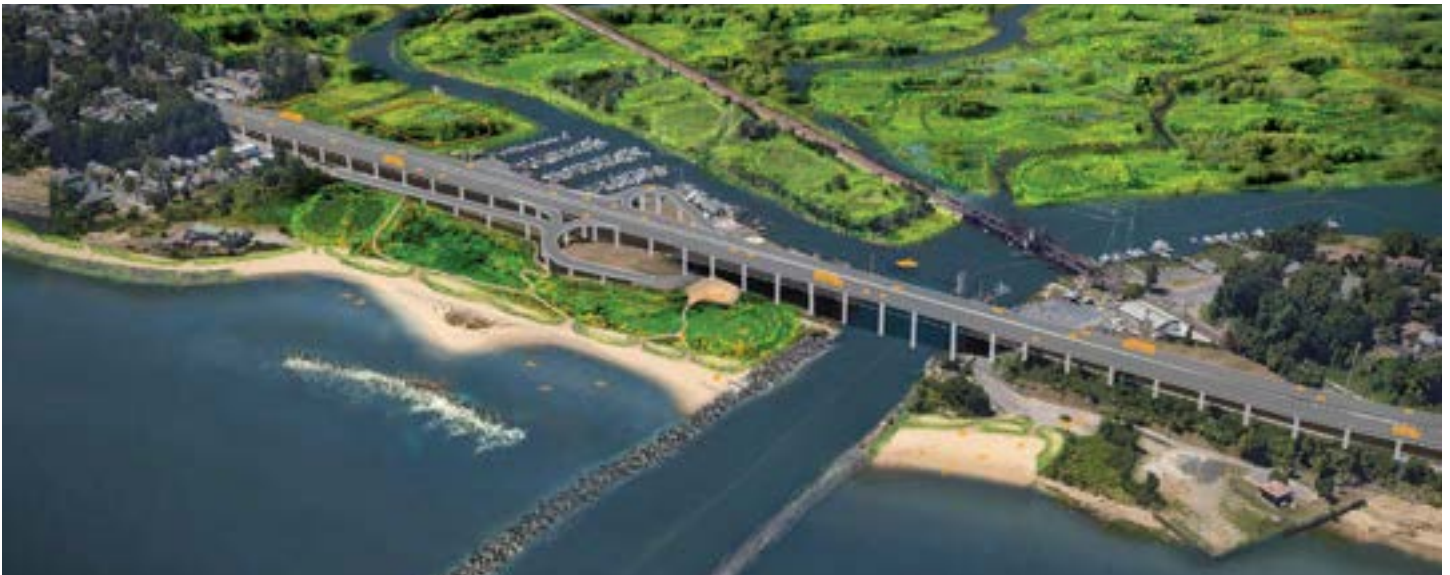
In Cheesequake Inlet, a multi-purpose flood barrier system is integrated into redevelopment sites on either side of Noe's Creek with living shorelines as a buffer.
