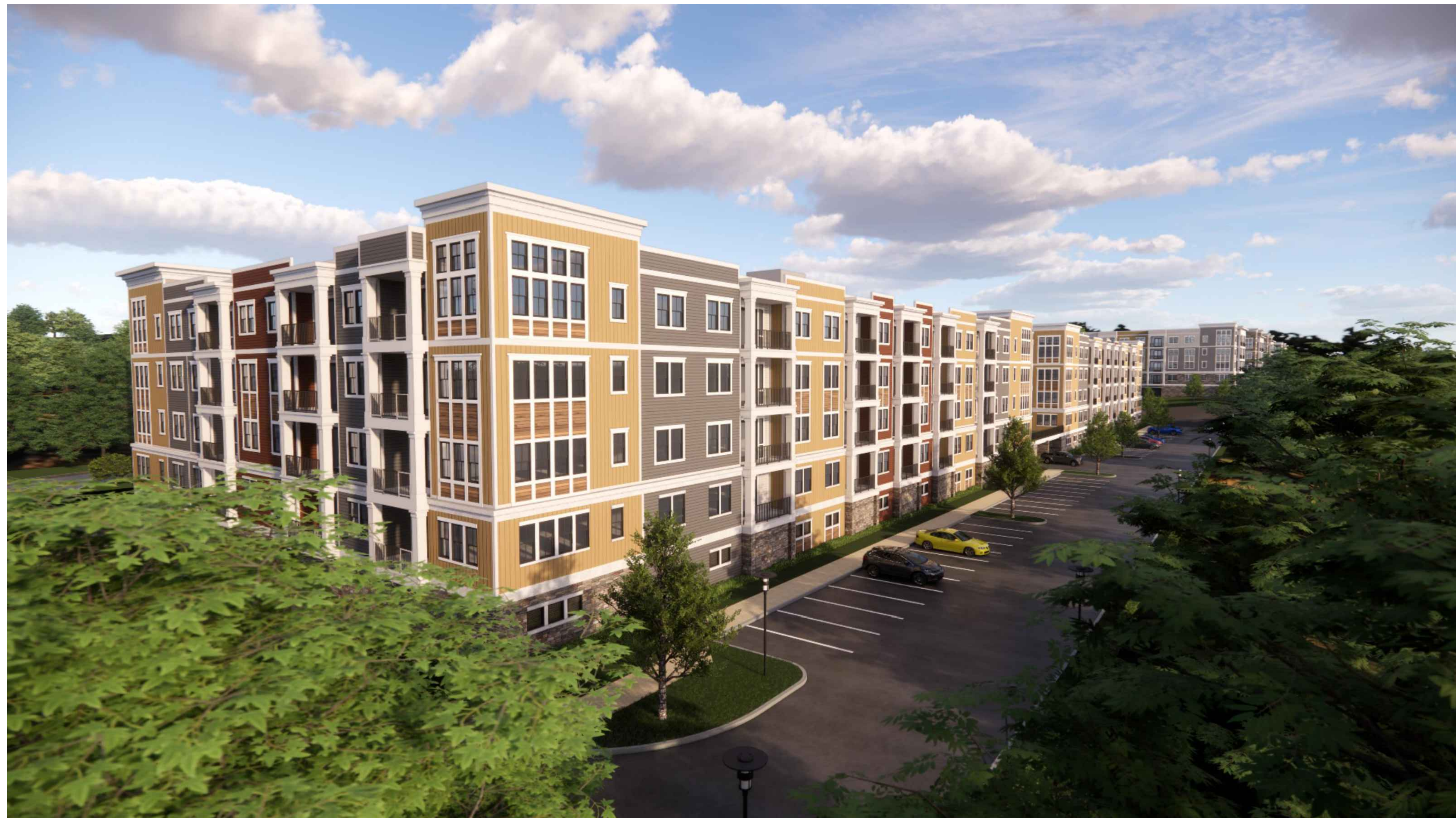
BUILDING 1 SOUTHEAST CORNER
