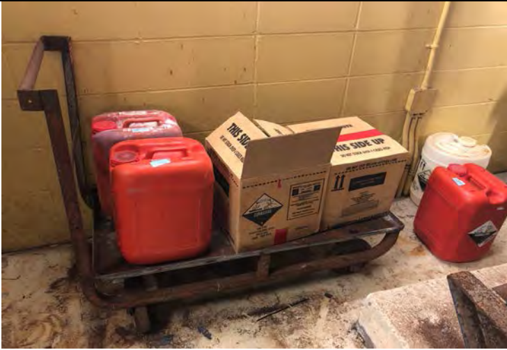
Photo 21: Containers of muriatic acid in pool mechanical room. Used for pool water treatment.
