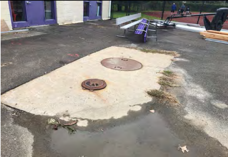
Photo 47: Active 1,000-gallon heating oil UST outside of the old vocational agricultural building.
