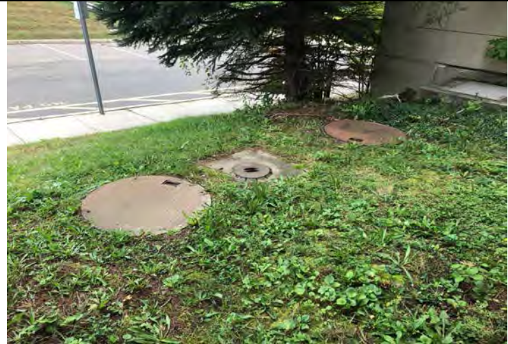
Photo 40: Inactive 6,000-gallon heating oil UST located outside of the new vocational agricultural building.
