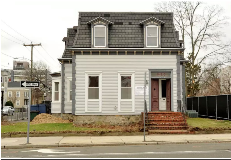
898 Summer Street circa 1875 (Northwest corner of Summer Street and North Street – This historic structure was demolished in 2014)
