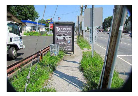
Transit shelter on High Ridge Road near Vine Street. Flooding, collection of mud and debris, lack of ADA access, lack of security (land use), and limited separation from moving traffic are a few of the problems with this shelter and transit stop.
