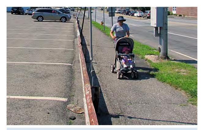
High Ridge Road near Cold Spring Road is just one area in Stamford where the guardrail has been placed at the back of the sidewalk. This is a significant comfort and safety issue for people walking or bicycling.
