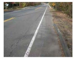
Typical pavement condition on High Ridge Road, between Merritt Parkway and North Stamford Road. Note the missing bituminous curbing on the right side of the road.
