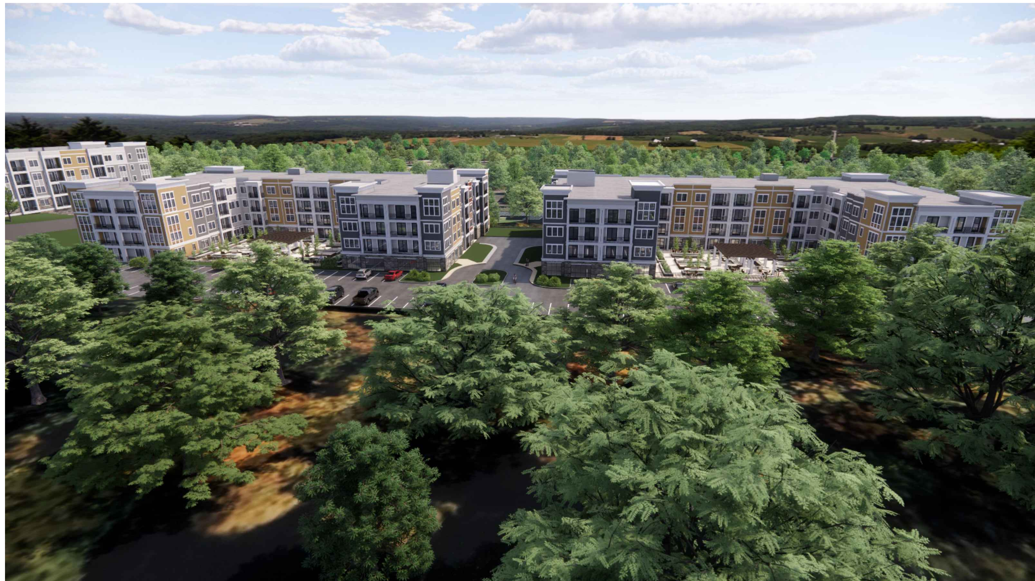
BUILDING 3 AND BUILDING 4 WEST FACADES
