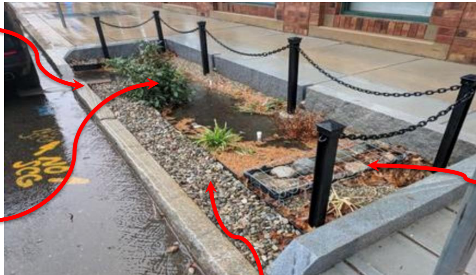
Sample Bioswale Rain Gardens – Photo(s) Courtesy of Yale School of the Environment Urban Resources Initiative
