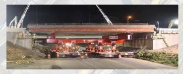
2. The old bridge will be demolished and the new bridge will be rolled into place on Atlantic Street. All tracks restored.
